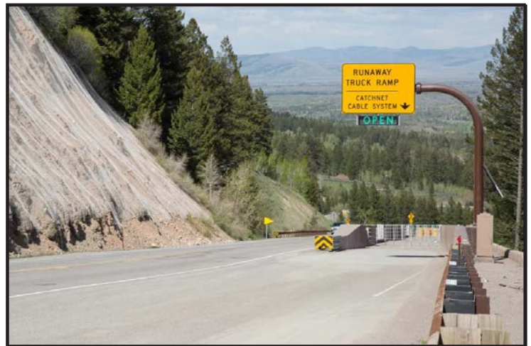
Image 2: Vehicle arrestor system at milepost 7.4 (buckrail.com)
