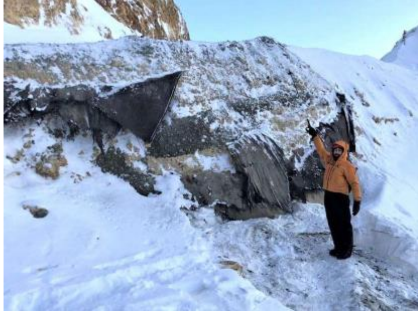
Figure 5. The same location as Figure 3 at the Pretty Rocks Landslide in January 2020 (National Park Service, 2020). The road had been displaced approximately 15 ft. since September 2019.
