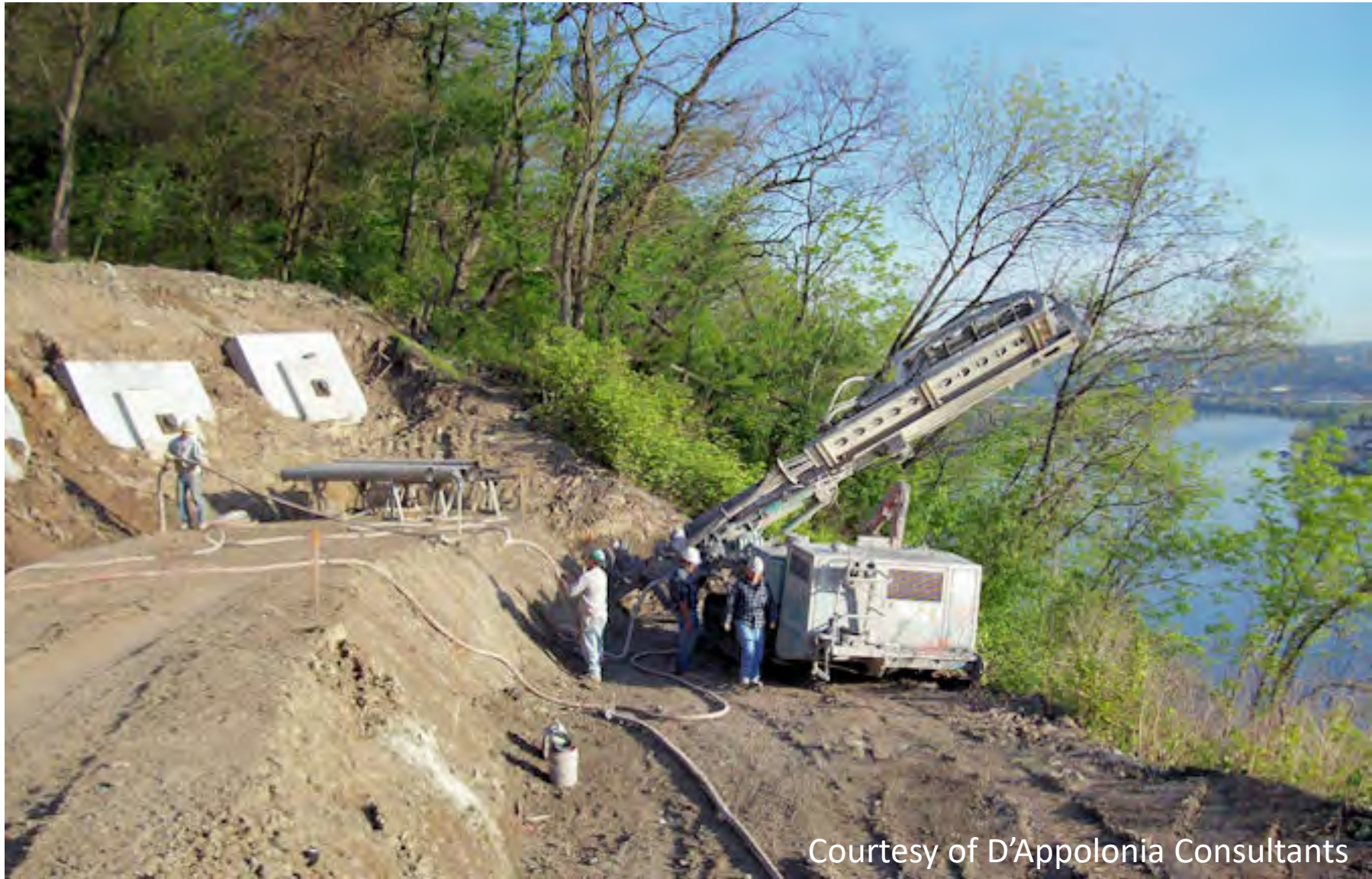
Figure 32. An example of high capacity anchors with bearing pads on the surface of landslide
