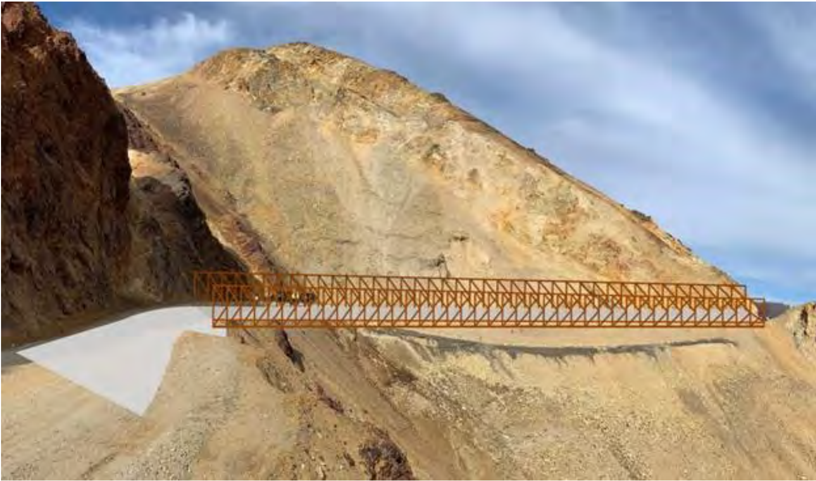
Figure 34. Rough concept of a modular steel truss constructed at Pretty Rocks Landslide, and the purple line on the LiDAR image to the right indicates the approximate bridge alignment and earthwork that would be required to accommodate the bridge option.
