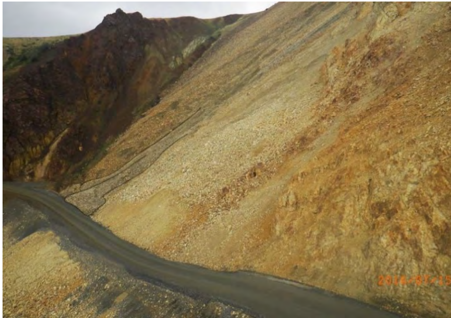
Figure 23: Two debris flows occurred on June 30, 2016. Partial outline of features highlighted for clarity. Road is one lane wide. Photo taken looking northwest.
