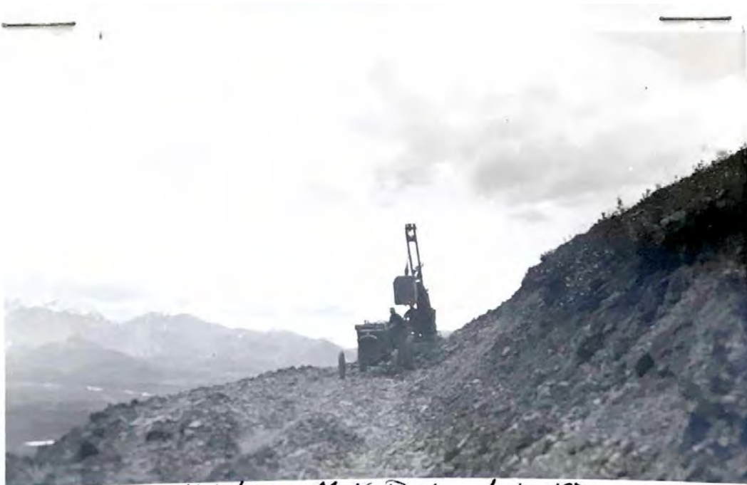
Grading High Line McK. Park July 1930
