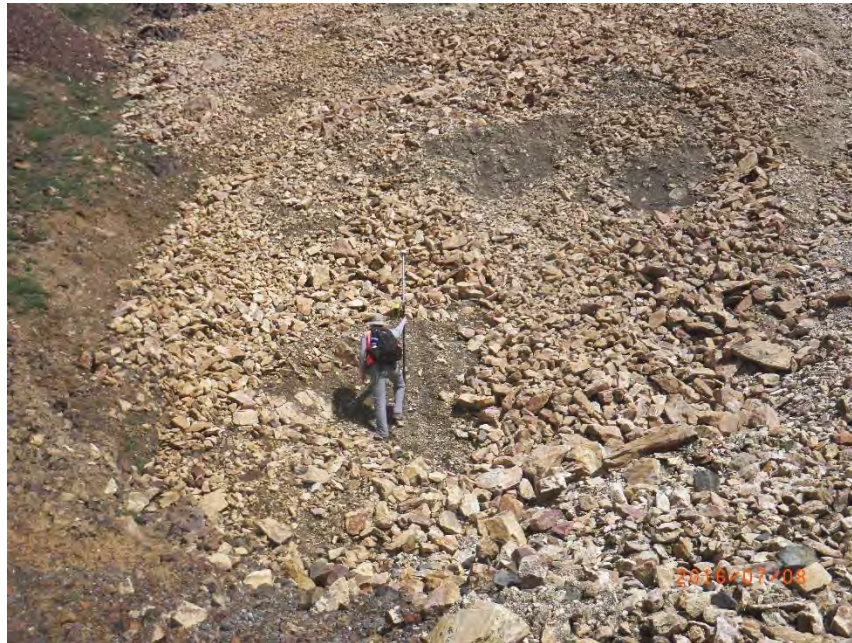
Figure 15: Outline of western boundary of failure area, and patches of slope devoid of cobble- to boulder-sized clasts. Picture taken roughly above the location of the western road crack.
