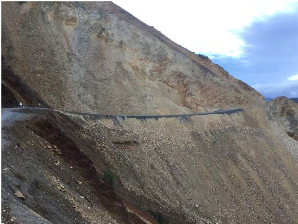
Figure 4-2. Denali Park Road at the Pretty Rocks Landslide. FHWA photo (2018).
