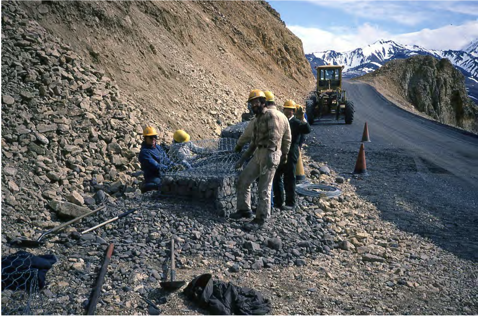
Figure 3. 1987 Installing Subsurface Drainage
