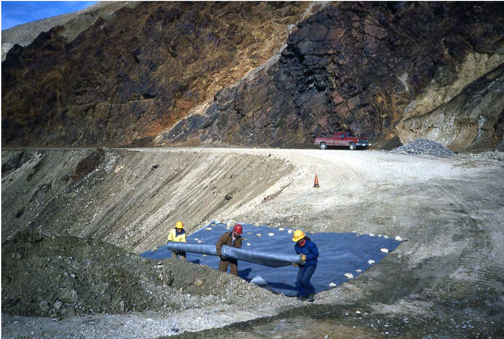
Figure 2. 1987 Installing geosynthetic layer reinforcement
