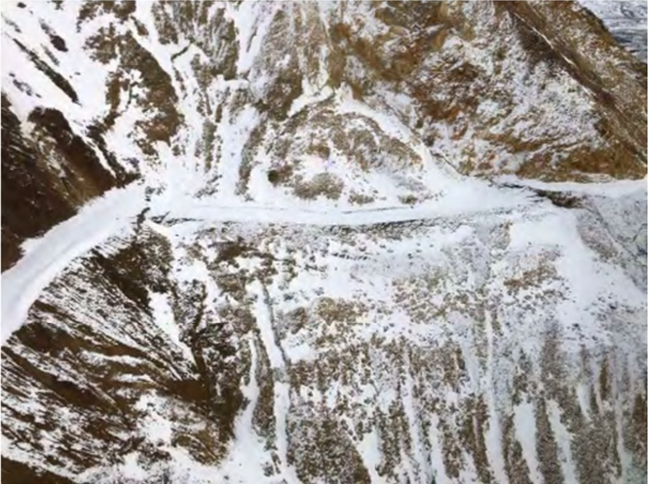
Figure 16: Aerial view of the Pretty Rocks Landslide area on the Denali Park Road from November 5, 2019 (Williams, 2019)
