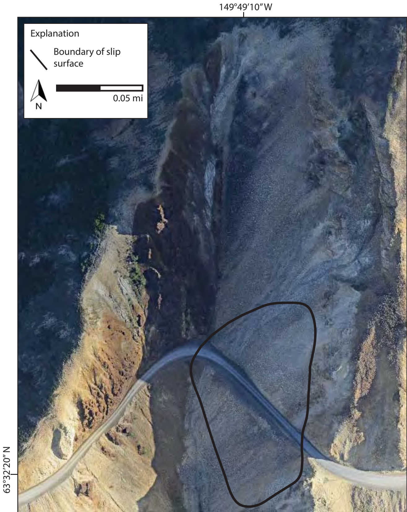
Figure 12: Proposed boundary of slip surface. Extent based on visual observations including cracks in talus slope, mapped locations of road cracks, crack dividing talus from rhyolitic bedrock to the east, and significant elevation changes seen in the Digital Elevation Model (Fig. 5).
