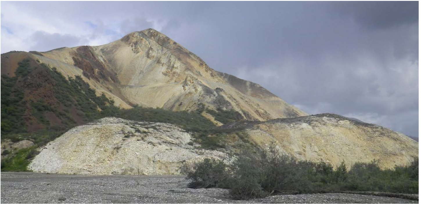
Figure 25: Pretty Rocks failure slope and lobe deposits seen from the East Fork Toklat River tributary. Photo taken looking north. Road visible in upper slope for scale.
