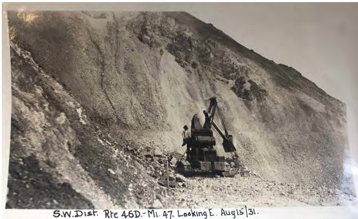
High Line Road being built in 1931 (Edmunds Collection, Box 1, Anchorage Museum)
