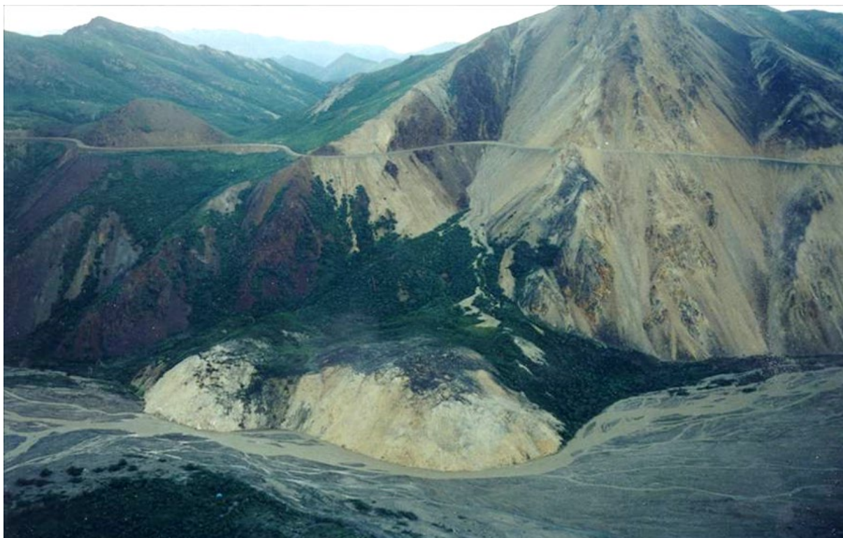
Figure 3-1. Denali Park Road at the Pretty Rocks Landslide. NPS photo (Date unknown).
