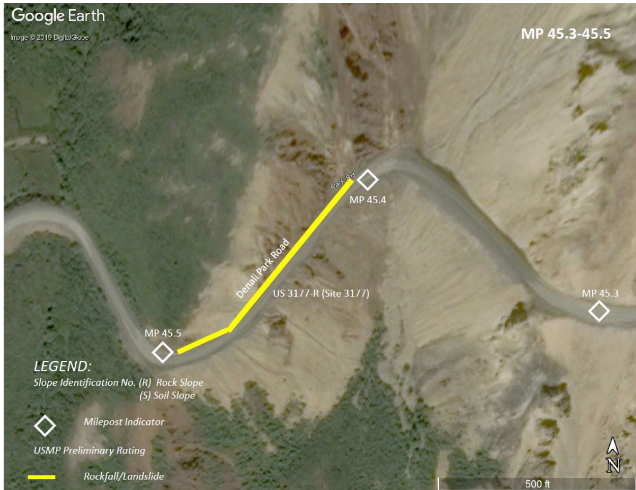
Figure 5-28. Overview of Sites 3177 between MP 45.41 and MP 45.48 on the Denali Park Road in Alaska (U.S Department of Transportation, December 2019).
