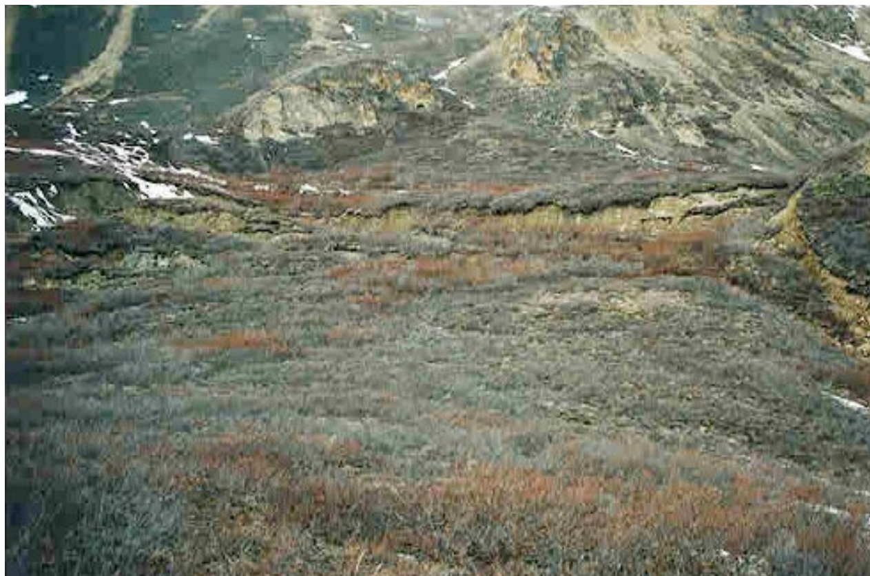
Figure 5-5. Looking upslope toward the MP 45 landslide headscarp from the lower center of the landslide.
