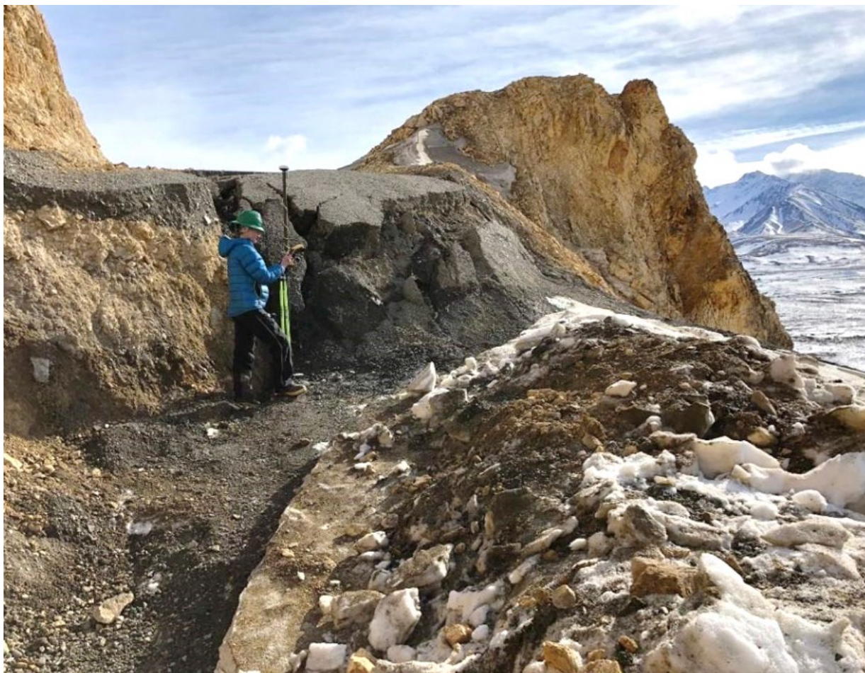
Figure 5-15. At the eastern Pretty Rock Landslide scarp. The area has fallen approximately 6.5 ft from September 2018 to when this photo was taken in March 2019 (NPS, 2020).
