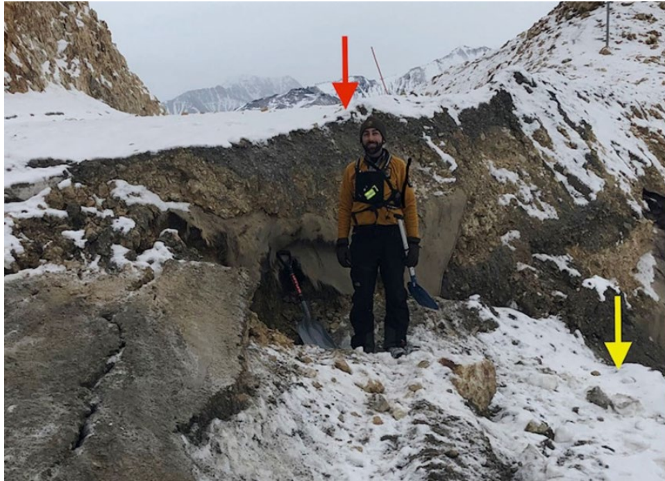
Figure 5-13. Pretty Rocks Landslide scarp at the Denali Park Road in November 2019 (NPS, 2020). The road had been displaced approximately 10 ft since September 2019 (from red arrow to yellow arrow).
