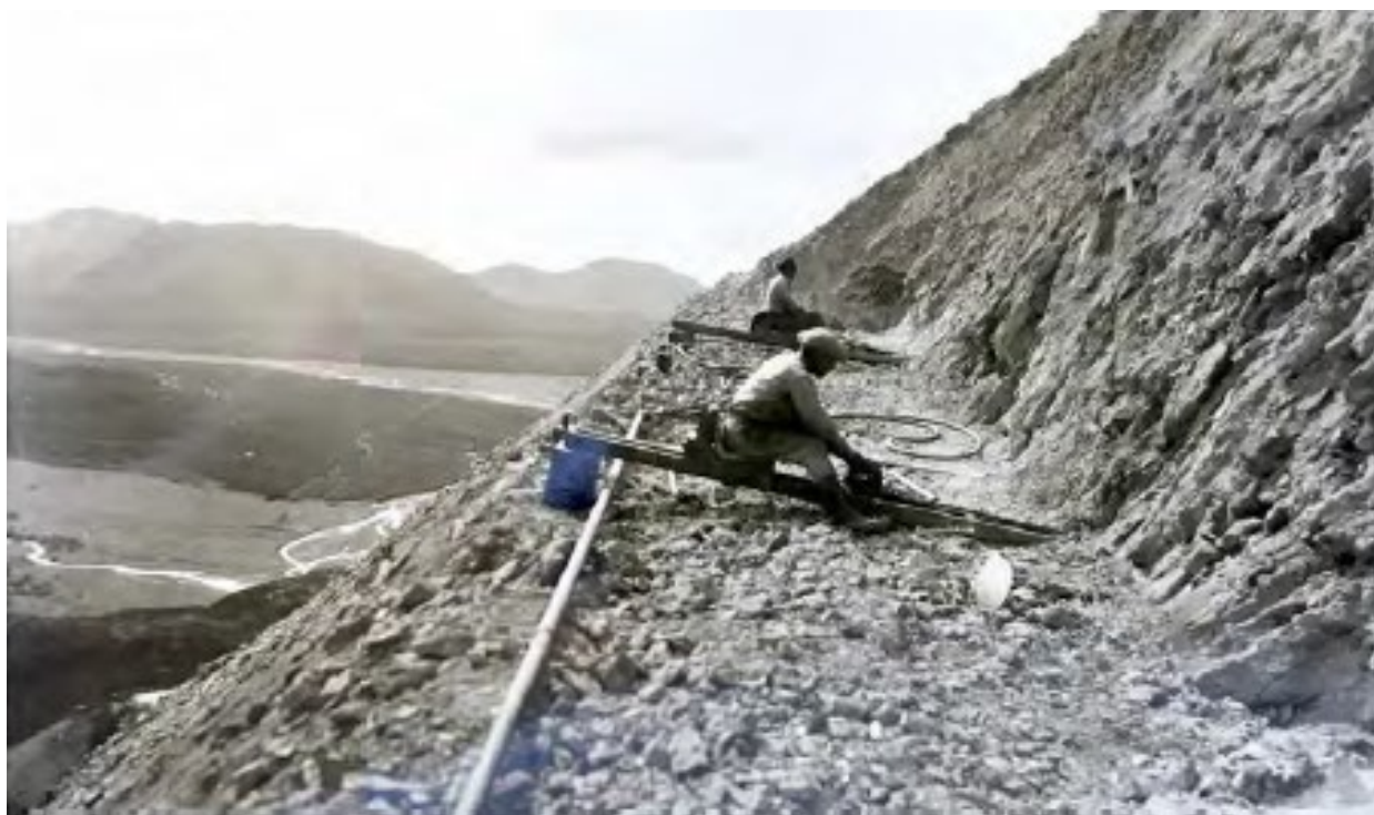
Figure 5-1. Drilling on the high line road, July 1930. (NPS, 2019).
