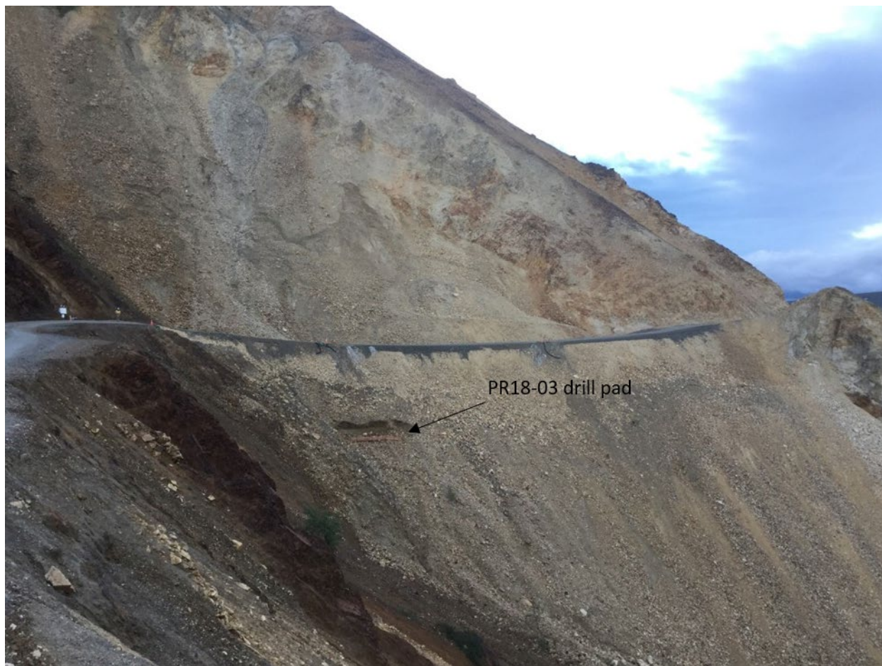
Figure 3-2. Denali Park Road at the Pretty Rocks Landslide. FHWA photo (2018).
