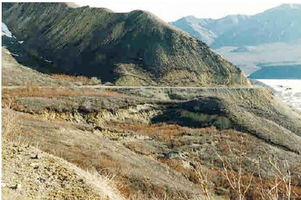
Figure 5-4. Looking east at the MP 45 (Bear Cave) Landslide from the west side of the landslide area in May 1996.
