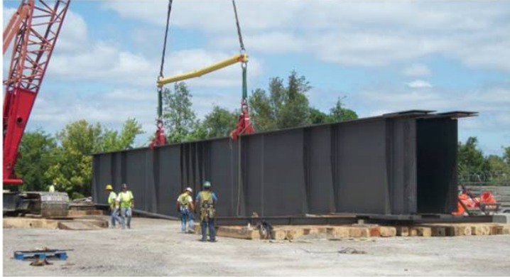
Figure 14: Storage of New Bridge Girders in Local Storage Yard
