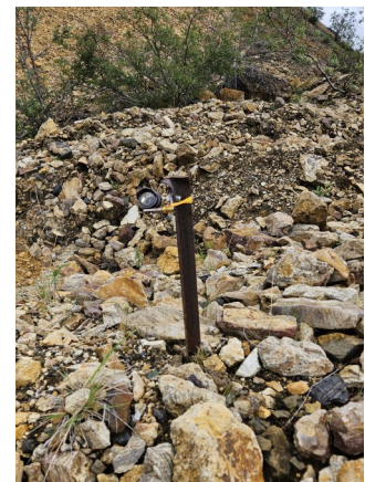
Geotechnical monitoring instrument installed.
