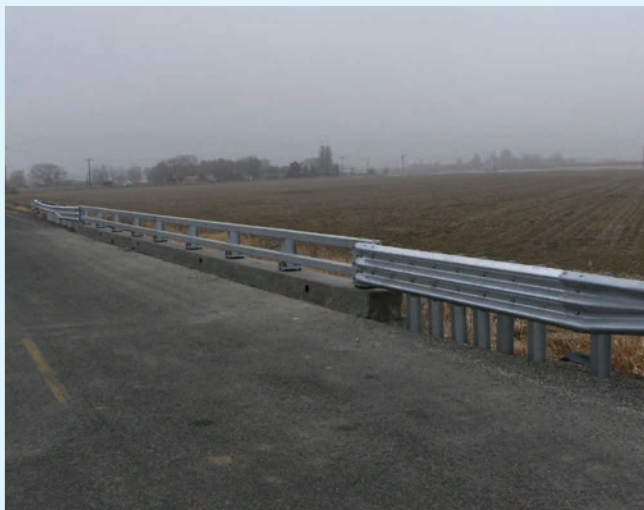
Bridge railing – example improvement resulting from the county safety program
