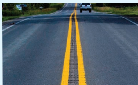
Centerline rumble strip in Michigan
