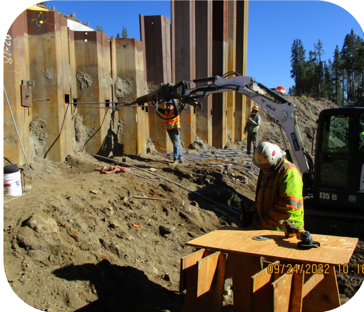
Installation of soil anchors.
