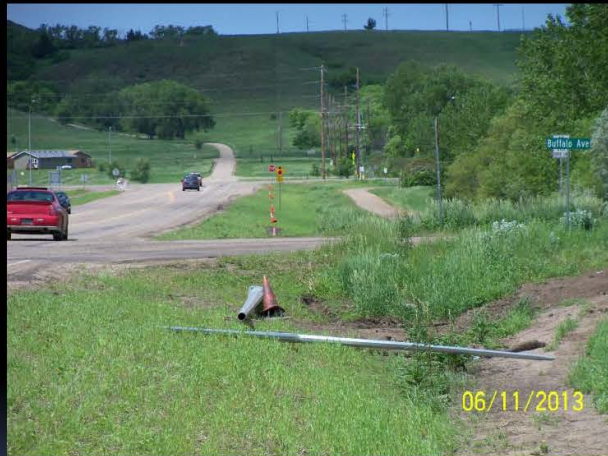
Lighting being put in on the walking path in Fort Yates
