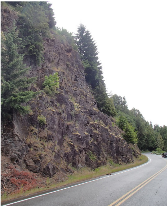
Figure 18. Rock cut where failure is controlled by interaction between geologic structure and rock friction. Forest Service Road 90, Milepost 13.
