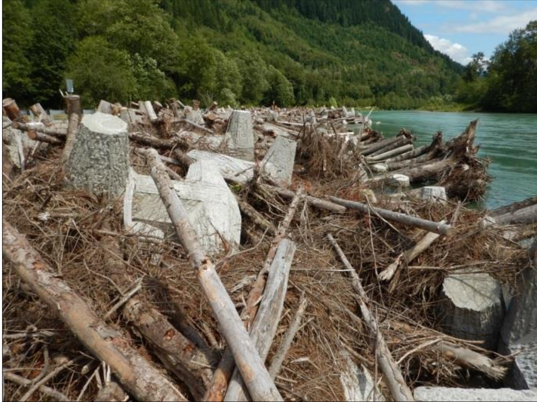
Figure 4-18. Typical ELJ/Dolosse Installation
