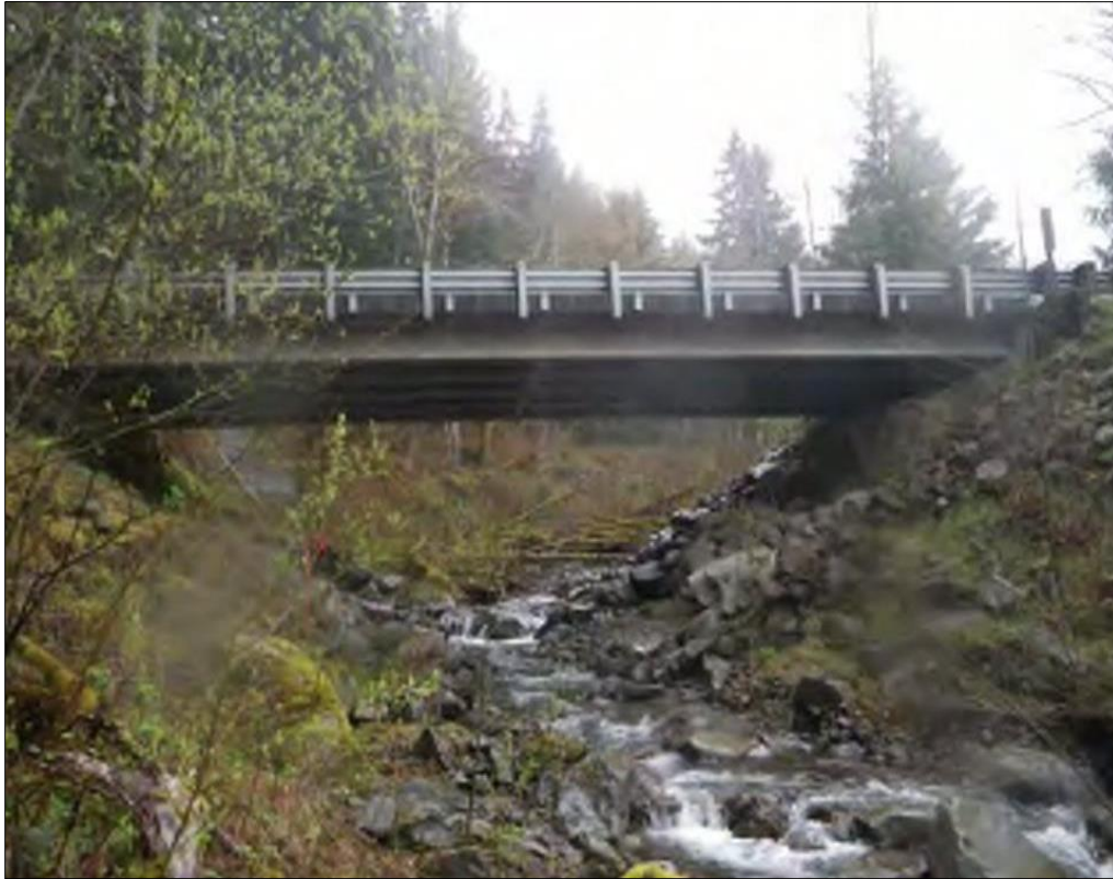
Figure 4-20. Tower Creek Bridge
