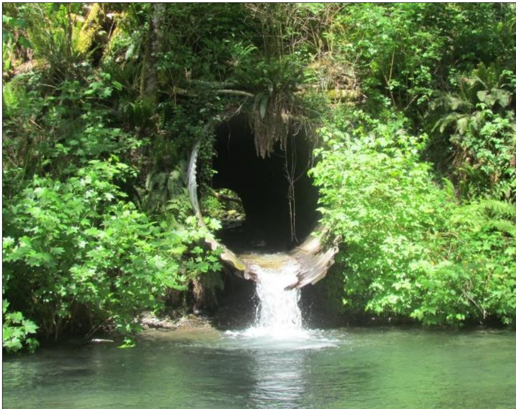
Figure 4-21. Canyon Creek Culvert
