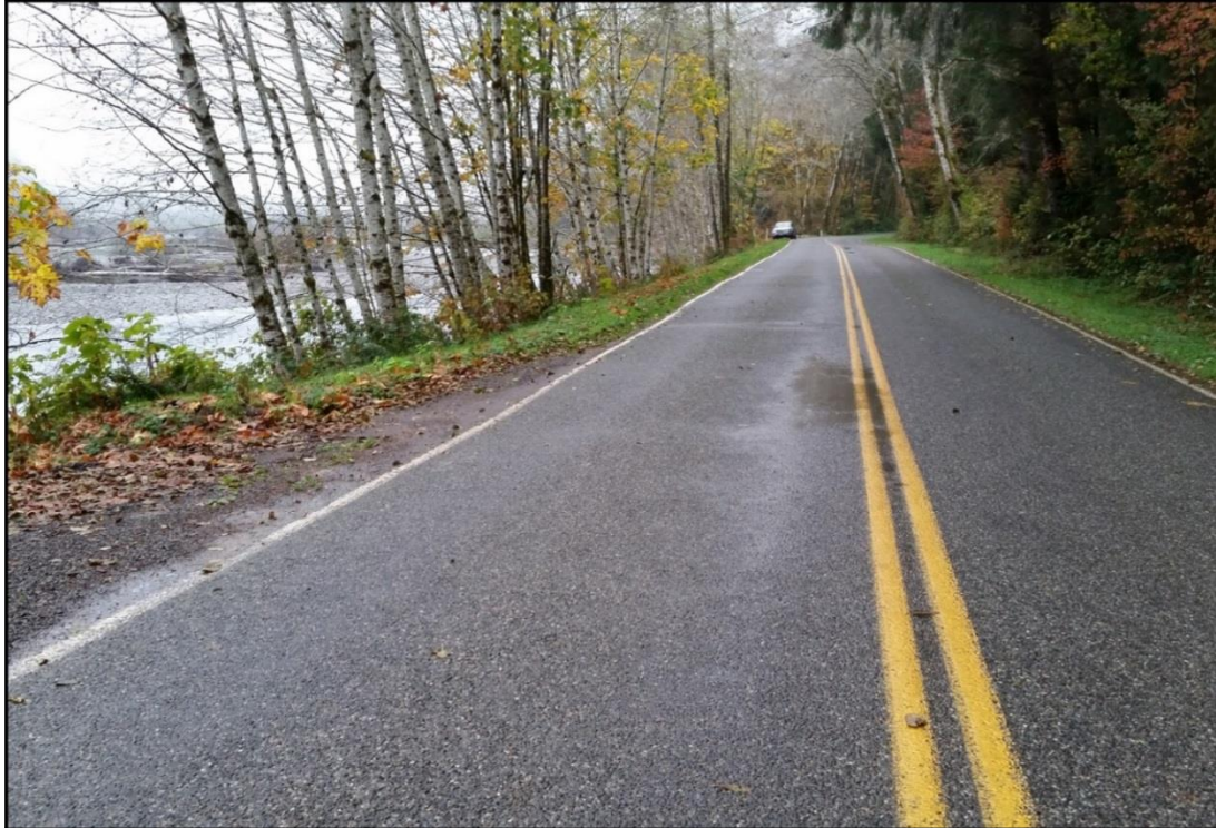
Figure 4-2. UHRR Typical Roadway Conditions
