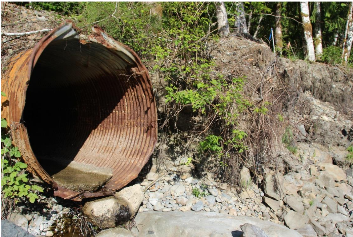
Figure 4-9. Existing Culvert at MP 4.38, Downstream End
