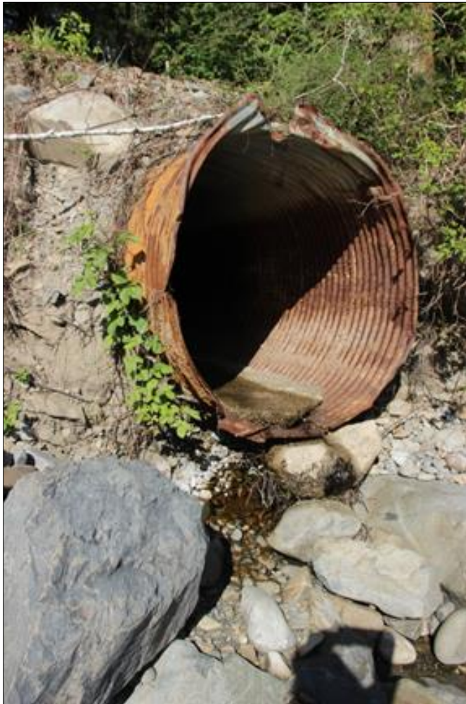
Figure 4-19. Existing MP 4.38 culvert to be replaced
