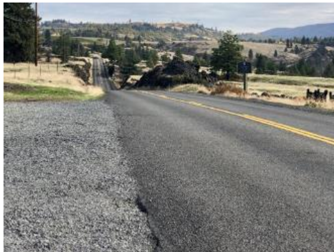
Facing east toward Catherine Creek Trailhead on south side of Old Highway 8
