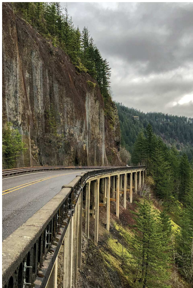
SR 14 through Cape Horn at the Western End of the Study Area
