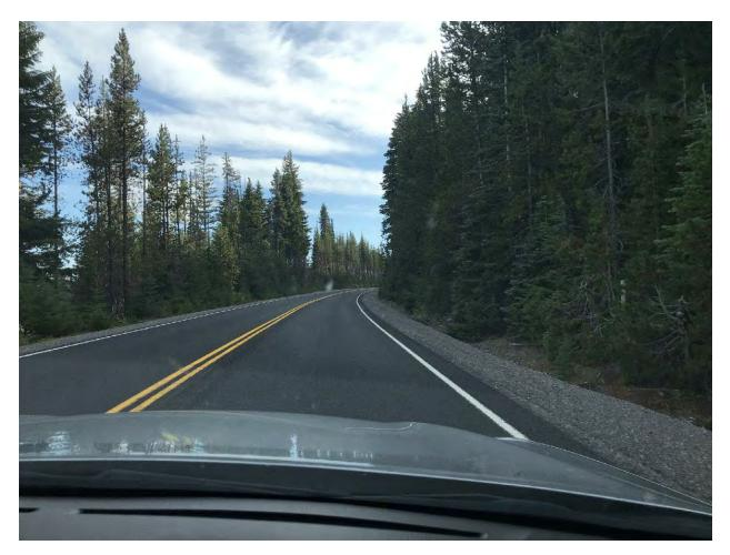
Figure 53 - Limited Horizontal Sight Distance in the Elk Lake Area
