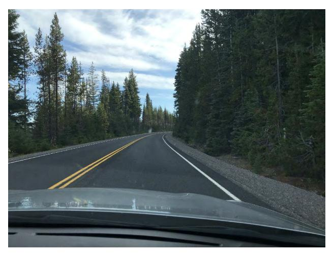
Figure 15 - Limited Horizontal Sight Distance in Section 6
