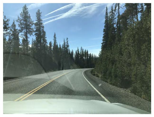
Figure 11 - Limited Horizontal Sight Distance
