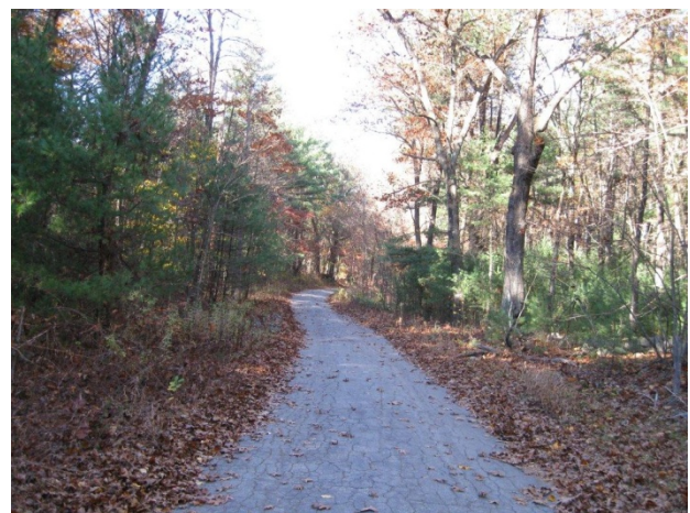
The recent project to construct a new parking lot at the North Entrance did not include repair of this 1,000-foot long roadway leading to the parking lot.
