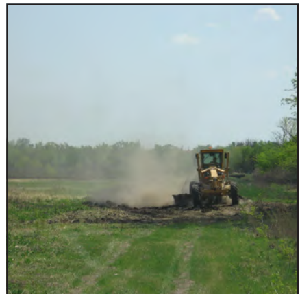
Road construction at Flint Hills NWR.
