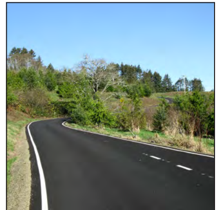
Curving roadway at Nestucca Bay NWR highlights scenery and discourages high speeds (top); emergency personnel respond to an accident at Ridgefield NWR (bottom).
