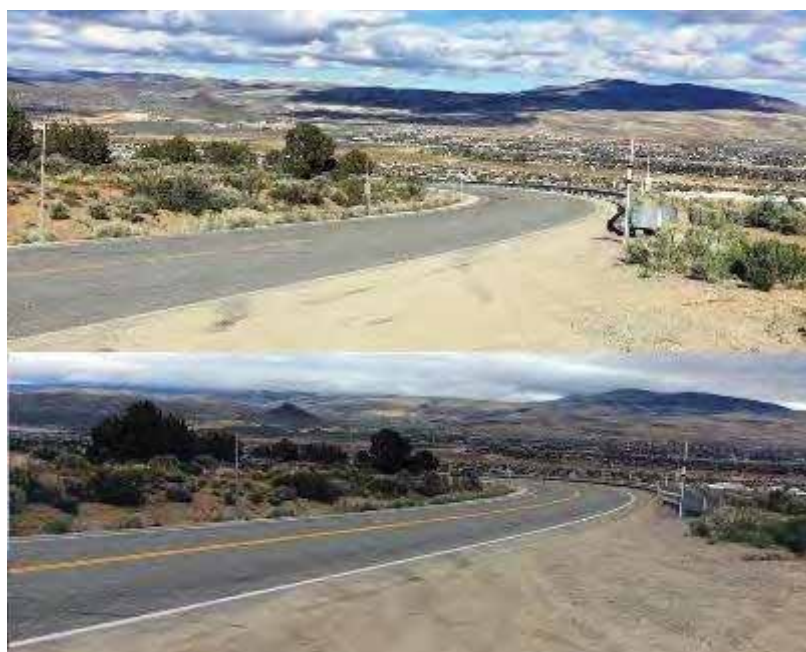
Figure 7. Before (top) and after (bottom) pavement marking maintenance by the Reno-Sparks Indian Colony Photo courtesy of Scott H. Carey, Reno-Sparks Indian Colony
