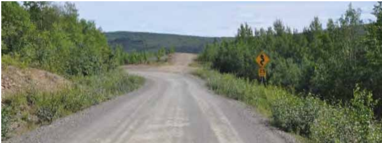
Figure 5. One third of roadway departure fatalities in Tribal areas occurred in a horizontal curve. Photo near the Native Village of Minto shows a visual trap that could lead a driver to miss the curve.
