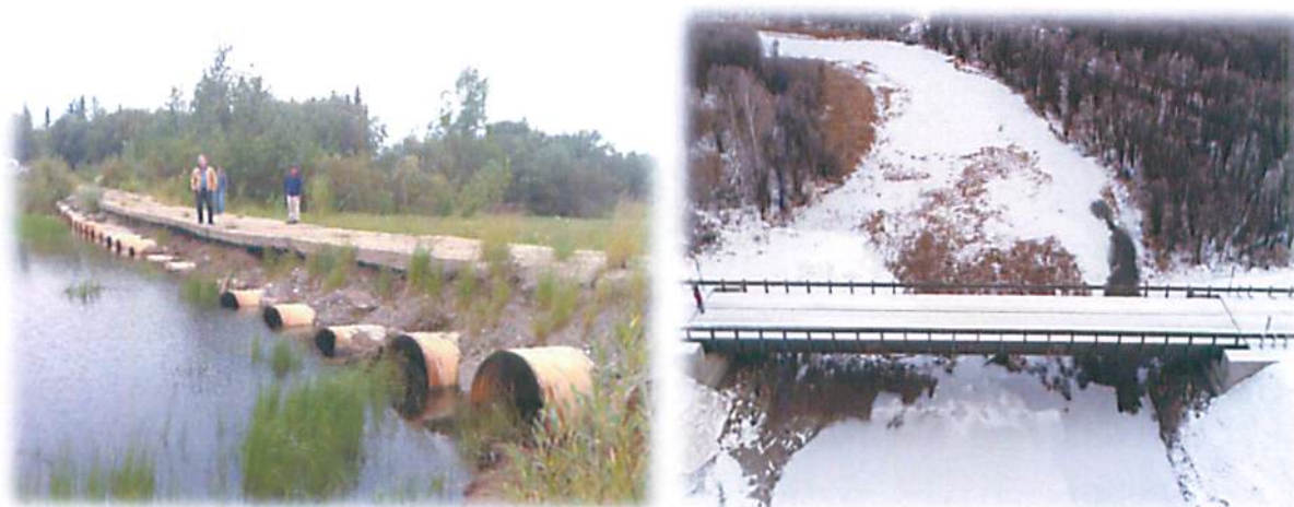
Ivar's Bridge Replacement Project (Before and After Photos), Fort Yukon, AK
