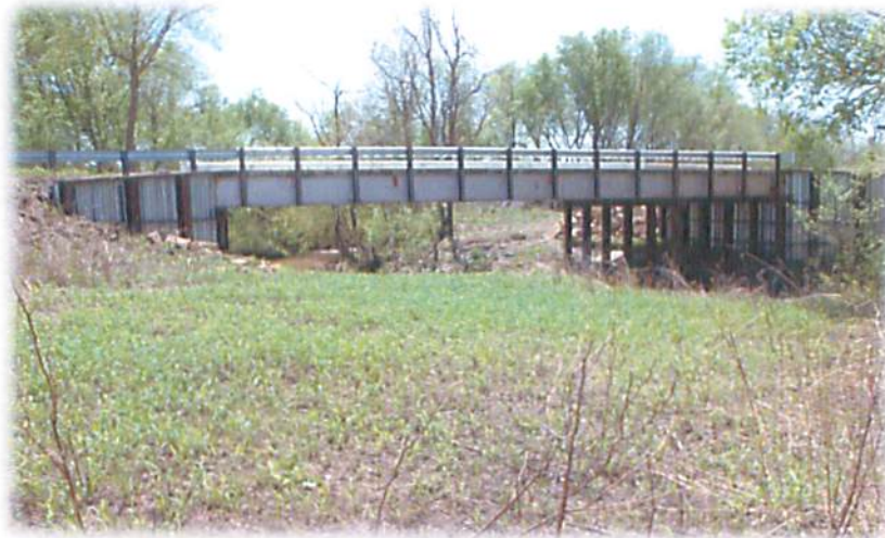
Bois D Arc Creek/Canteen Road, Kay, OK
