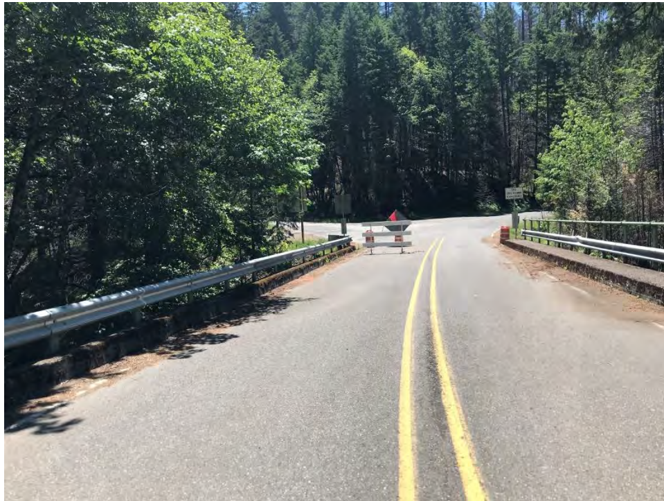
Figure 5: Apparently Undamaged Guardrail and Bridge Rail (OR 224, MP 49.97)
