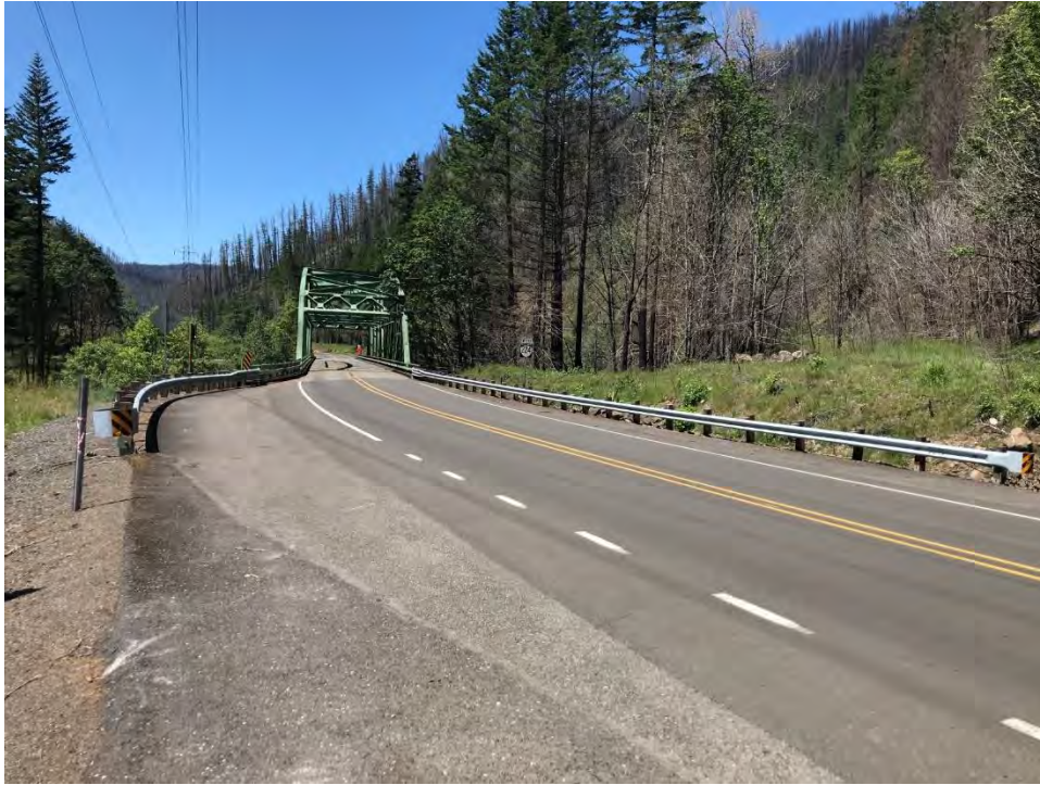
Figure 4: Apparently Undamaged Guardrail and Bridge Rail (OR 224, MP 31.2)
