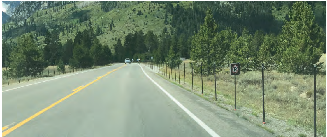
Grand Teton NP- delineators with No Parking symbol signs along shoulder
