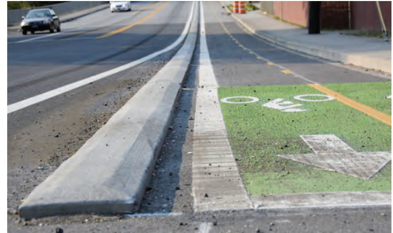
Low-profile curbs being used to separate traffic modes
