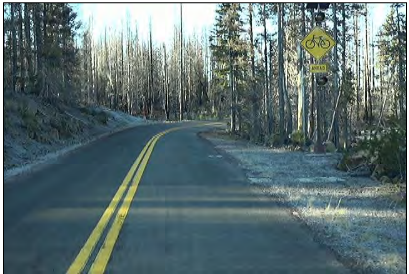
Figure 3: Dynamic Warning Sign for Bicycles (OR 242, MP 78.6, ODOT Digital Video Log)
