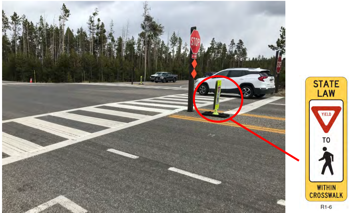
Figure 3: High Visibility Crosswalk Markings with In-Street Signage (Yellowstone National Park; installation along OR 224 likely not in stop-controlled areas)
