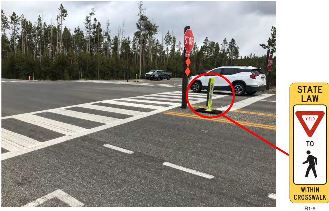
Figure 5: High Visibility Crosswalk Markings with In-Street Signage (Yellowstone National Park; installation along OR 224 likely not in stop-controlled areas)
