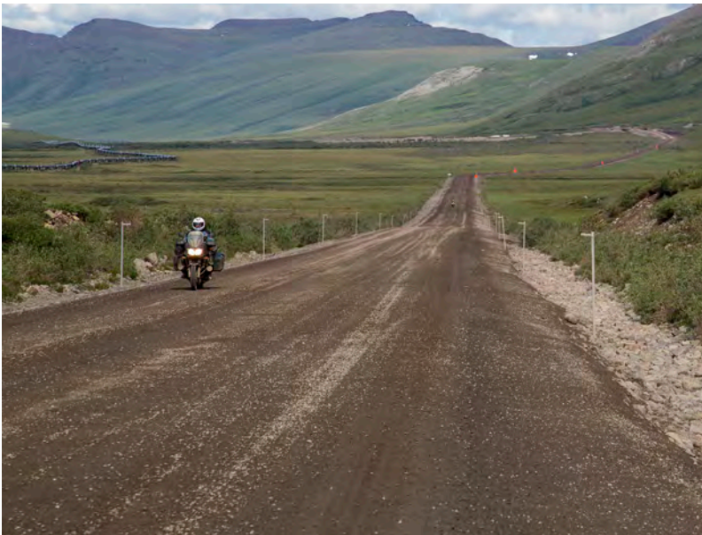
Dalton Highway (Roadway Vulnerable to Permafrost Thaw). BLM photo.
