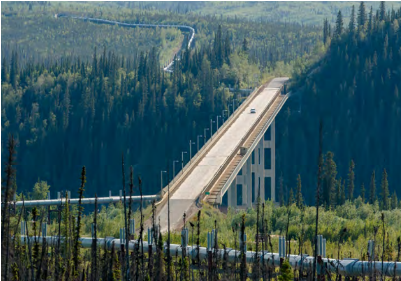
Dalton Highway Crossing the Yukon River. BLM photo.
