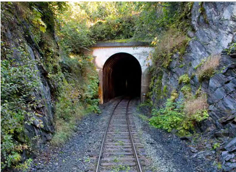
Chugach National Forest, Alaska Railroad Glacier Discovery Train Tunnel. FS photo.
