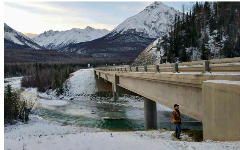
Bridge Inspection. Alaska DOT&PF photo.
