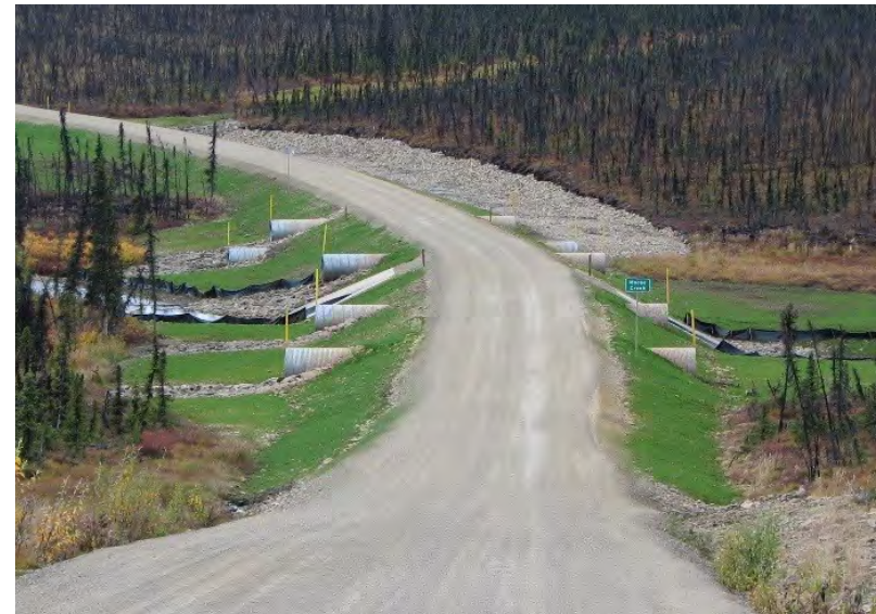
Culverts at Nome Creek, White Mountain National Recreation Area. BLM photo.
