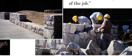
Stonemasons fit the shaped stones together and apply mortar. Inset: Completed stone wall at Fife's Peak Overlook. Photos courtesy Gary Hunter
