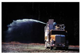
A hydroseed truck shoots a mixture of water, grass seed, fertilizer, and mulch over the topsoil on the reclaimed borrow pit. Photo courtesy Gary Hunter
