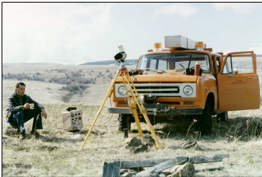
Ted Breneman lets his equipment do the work during a 1973 survey. WFLHD Archives.
