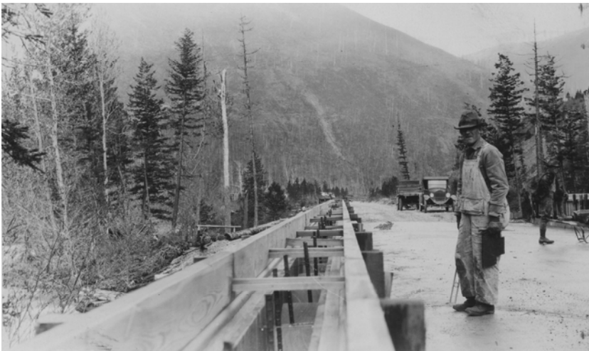
The Final Construction Report on the project at Columbia Falls-Glacier Park in the 1920's described this photo as “Handrail forms, Bear Creek # 3. These forms were built in 16 foot panels with staggered joints.” H. A. Stoddart, Jr., was the Civil Engineer who submitted the report. WFLHD Archives, 1920's construction.
