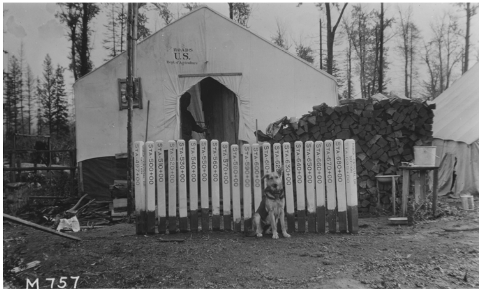
Final Construction Report on Columbia Falls-Glacier Park Project (Formerly Belton-Java) Nyack-Crystal Creek Station (1923-1924-1925) shows “Maintenance stakes carved with a jack-knife.” The report was submitted by E.E. Avery, Chief of Road Survey Party.
