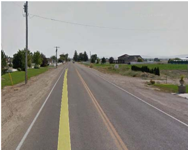
Midway Road & Orchard Ave (south, 24ft wide)
