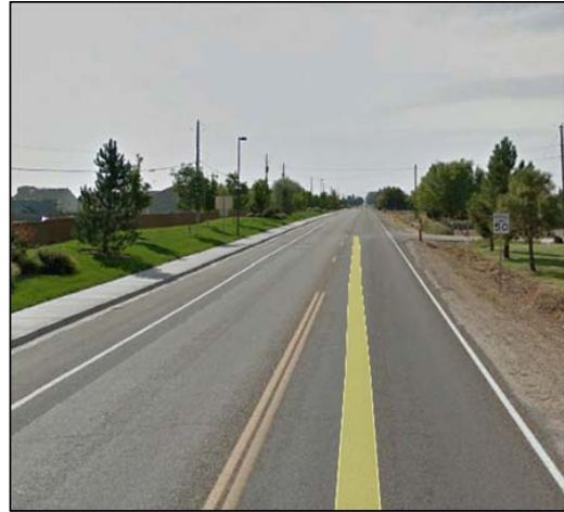
Lake Ave & Karcher Road (south, 24ft wide)
