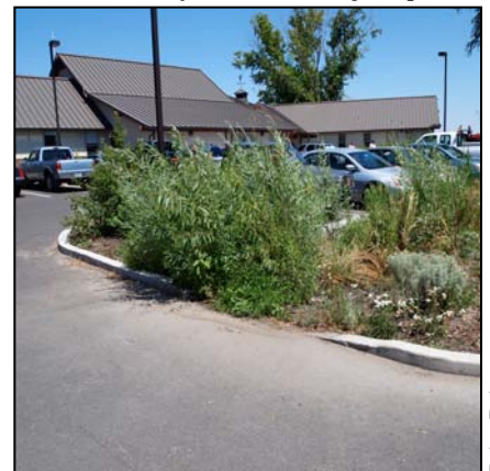
Parking lot runoff at McNary NWR drains to a central bioswale that treats polluted runoff and buffers habitat from roadway impacts.
