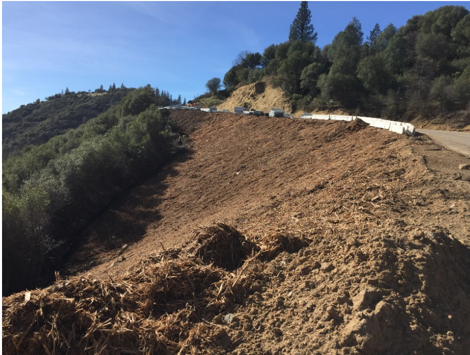
Figure 33: Wood Slash/chips blown on slope for temporary or permanent mulch.
