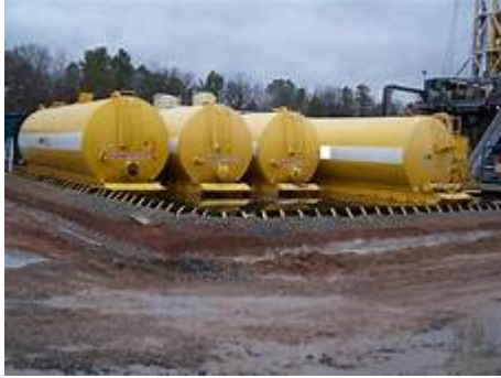
Containment berm around tanks
