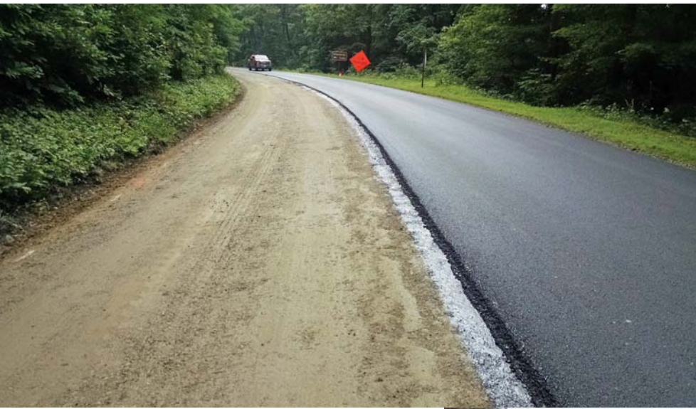
Left: Part of freshly surfaced ½ lane-mile.
