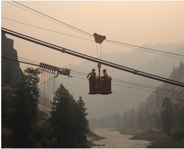
Workers brave the heights to attach cables which will provide stabilization to the bridge
