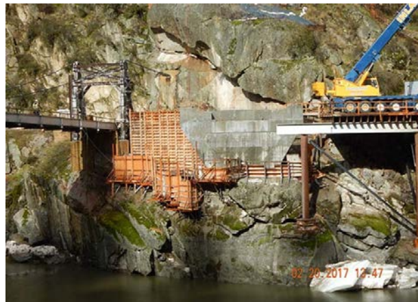
Concrete support form for Steel Tower
