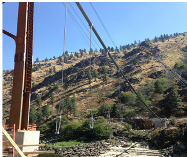
Workers brave the heights to attach cables which will provide stabilization to the bridge
