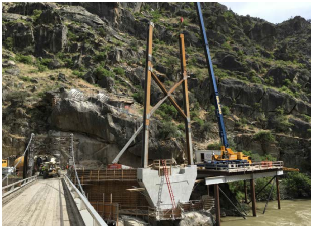
The 75 ft Steel Tower erected on the north end
