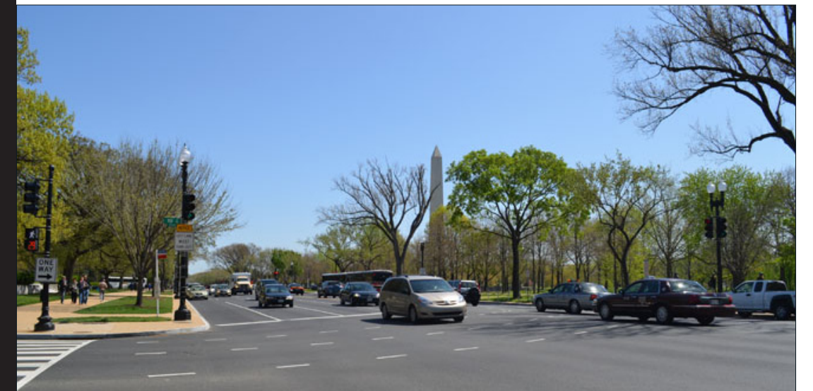
Urban Streetscape Improvements, Rehabilitation, ADA compliance
