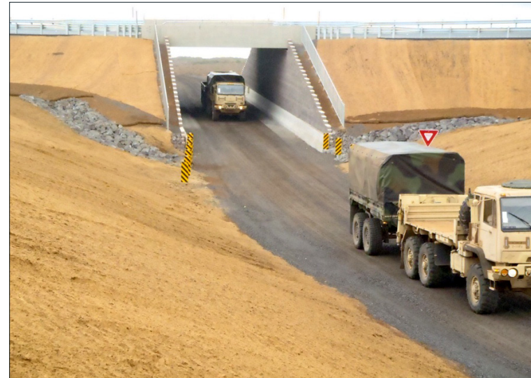
GRS-IBS Bridge under Saddle Road provides military operation access.
