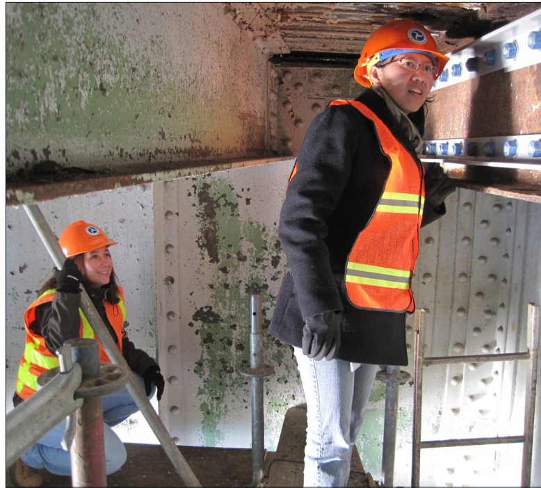
Construction & Structural Engineers Conducting Bridge Inspection
