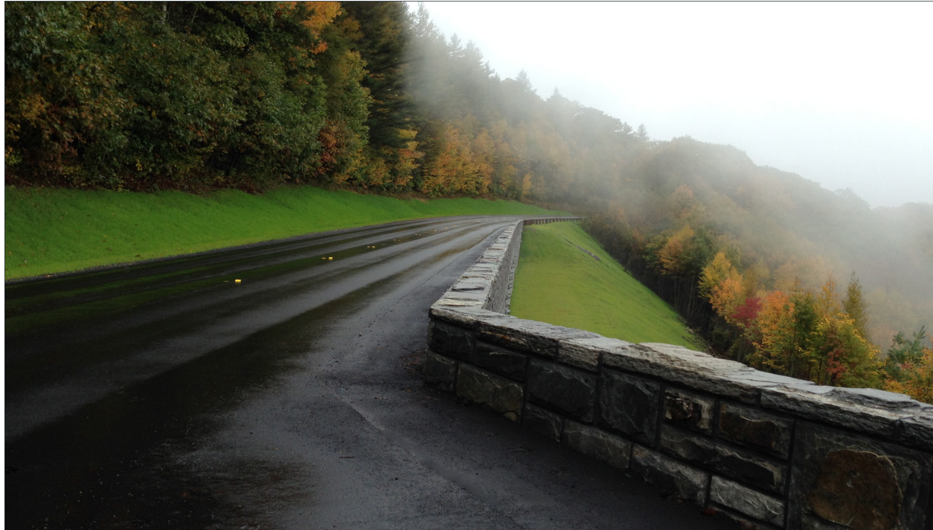
Slide Repair, Value Engineering, Innovative Contracting
