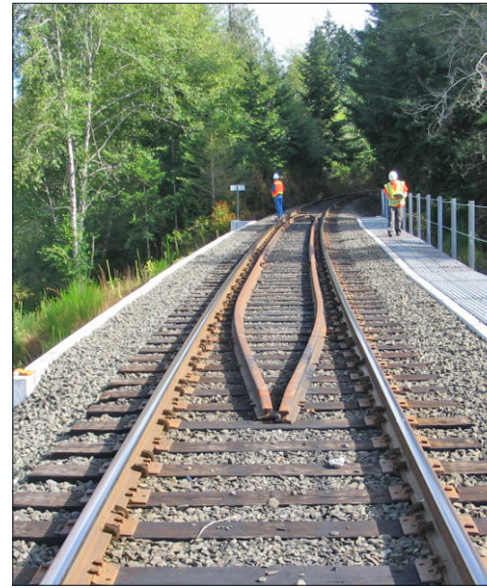
Railroad Bridge Inspection
