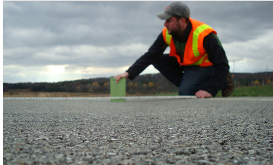
Pavement Engineer Measuring Asphalt Pavement Rut Depth
