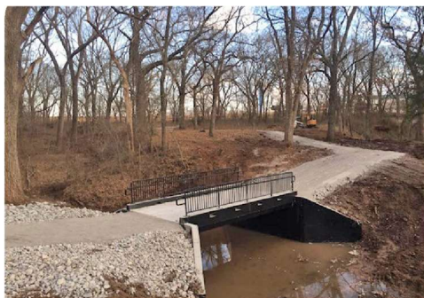
Pawnee Nation ICDBG Ceremonial Campgrounds and Nature Fit Trail Project was the 2nd to use a “Fast Cast Bridge” system and the 1st to use a “Fast Cast Bridge” system for a Pedestrian Bridge. — Pawnee, Oklahoma
