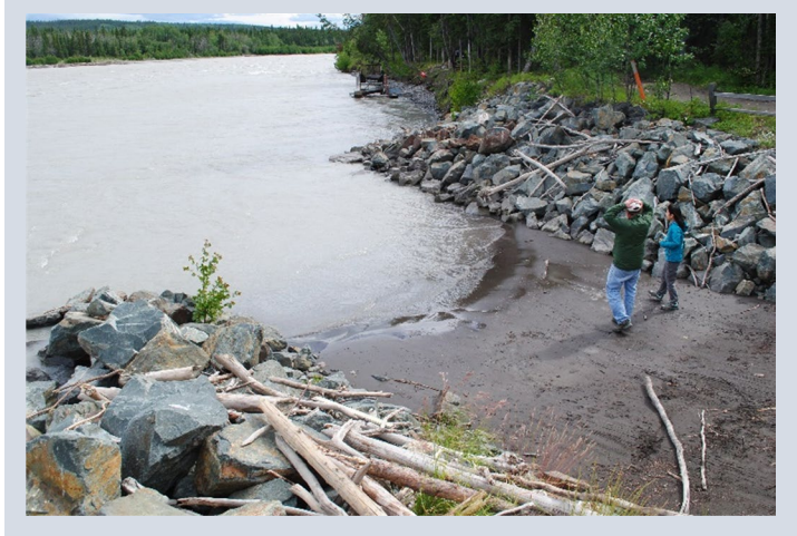
Figure 12. Copper Center private boat launch.
