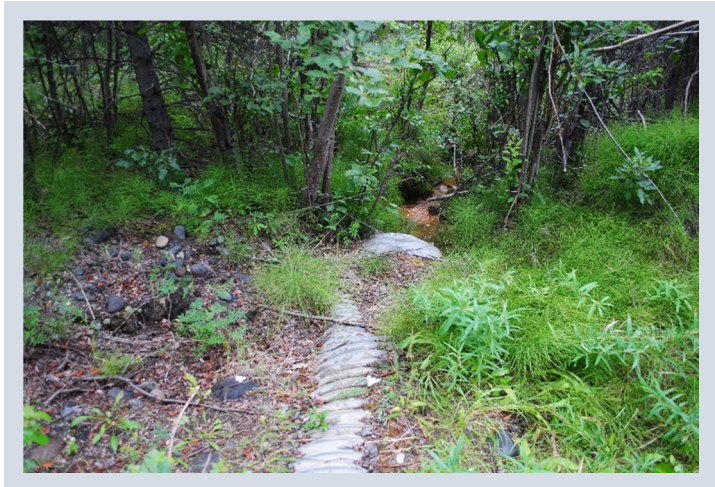
Figure 13. Culvert in project area.
