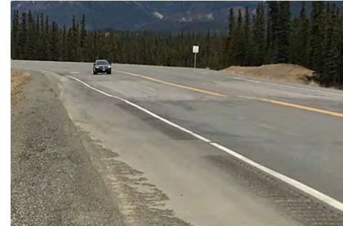
Annual pavement maintenance (~MP 232.7)
