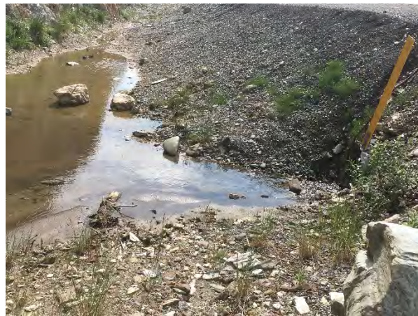
Figure 57. Upstream Side of Culvert Looking South Near MP 241
