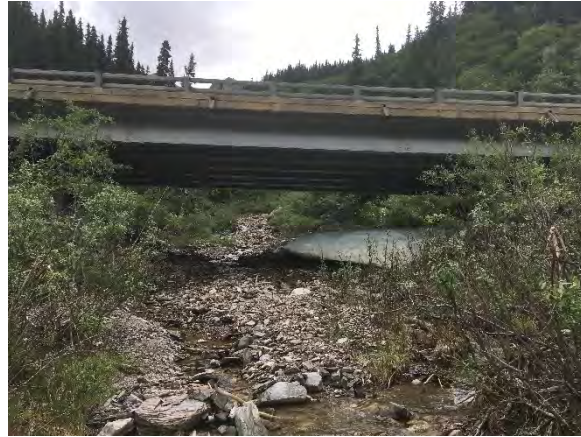
Figure 26. Fox Creek Bridge (BR 1144), Upstream Looking Downstream
