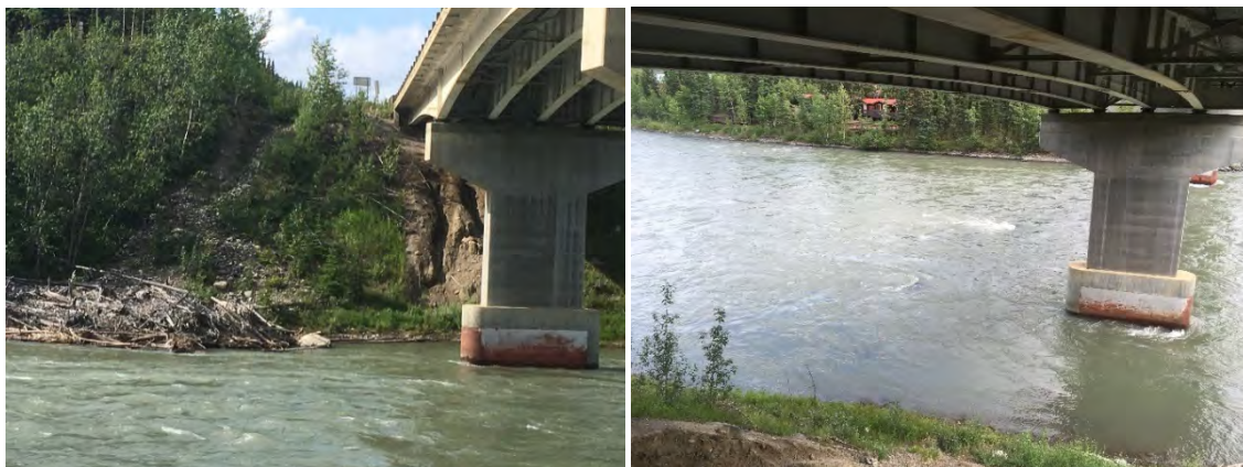
Figure 13. Looking Upstream, At Left Abutment, Looking Upstream from Left Abutment
