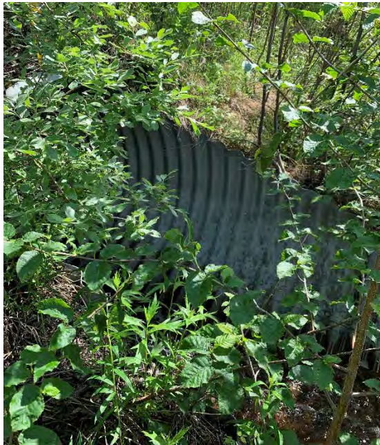
Figure 25. Grizzly Creek Cross Culvert, Upstream Side Looking North
