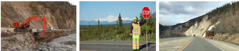
Example photos of roadway construction and rock fall hazards.
