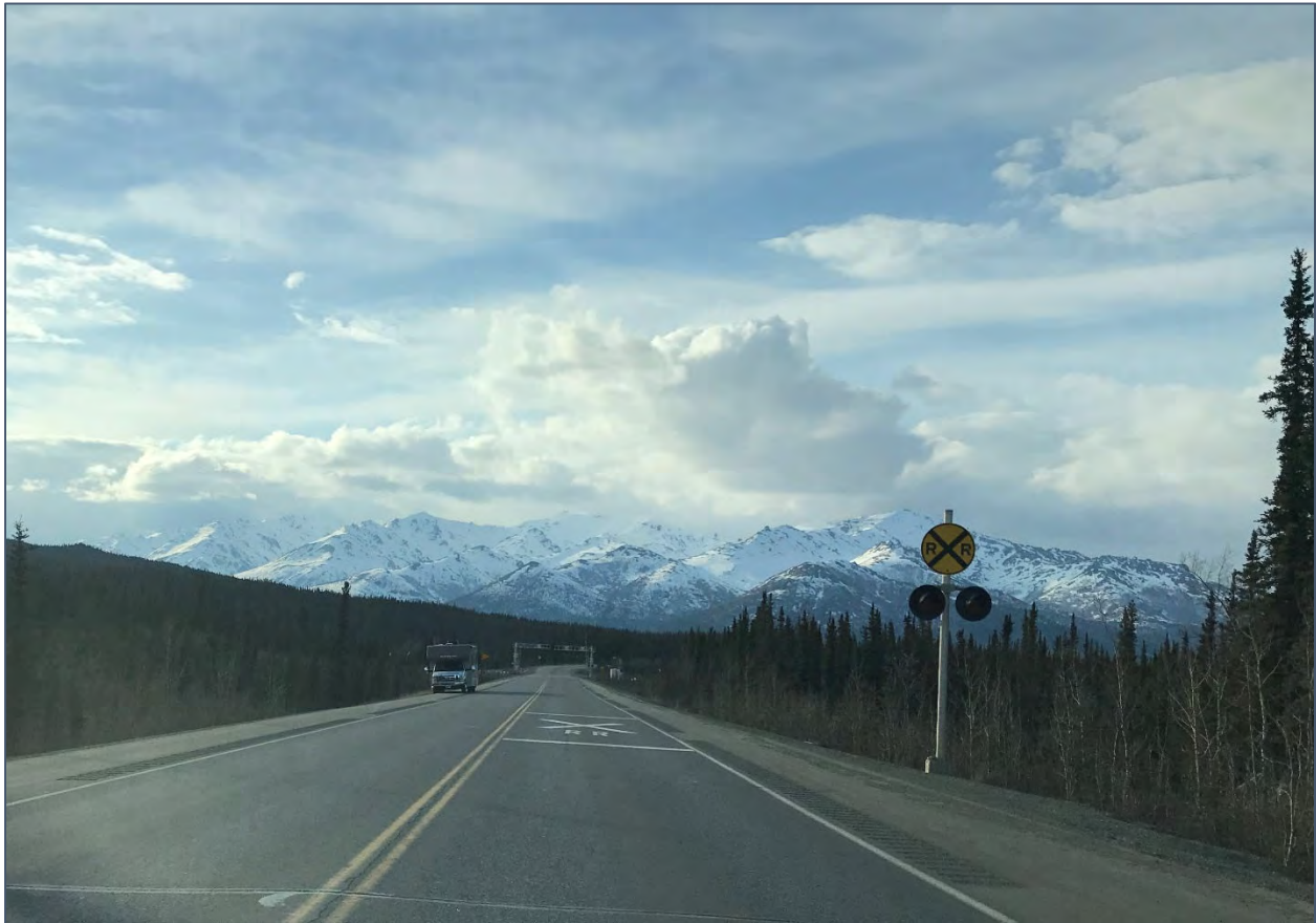
Image of at-grade crossing at Parks Highway MP 235/ ARRC MP 345, looking northbound.
