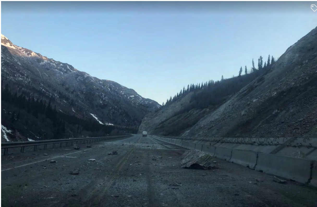
Figure 17 – Larger rockslide that has traveled onto the Parks Highway in Nenana Canyon
