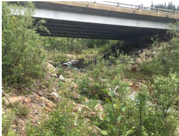
Figure 23. Hornet Creek Bridge (BR 1145), Downstream Looking Upstream
