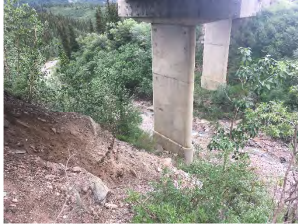
Figure 37. Antler Creek Bridge (BR 1141), Downstream Looking Upstream and East
