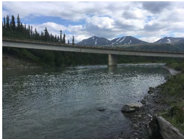
Figure 6. Nenana River Bridge (BR 1243) Downstream Looking Upstream
