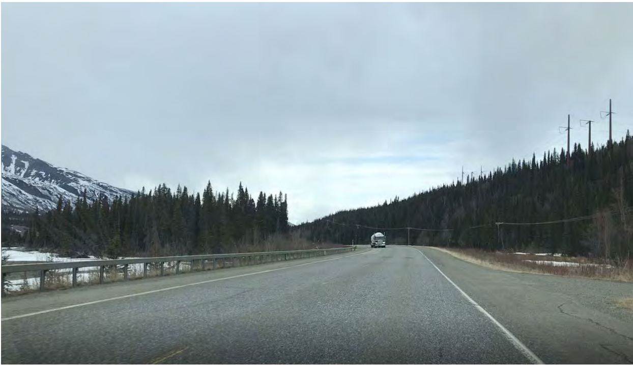
Roadway curvature with Nenana River abutting highway, south of MP 223
