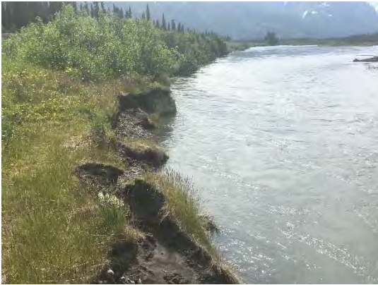
Erosion just north of MP 223 looking south
