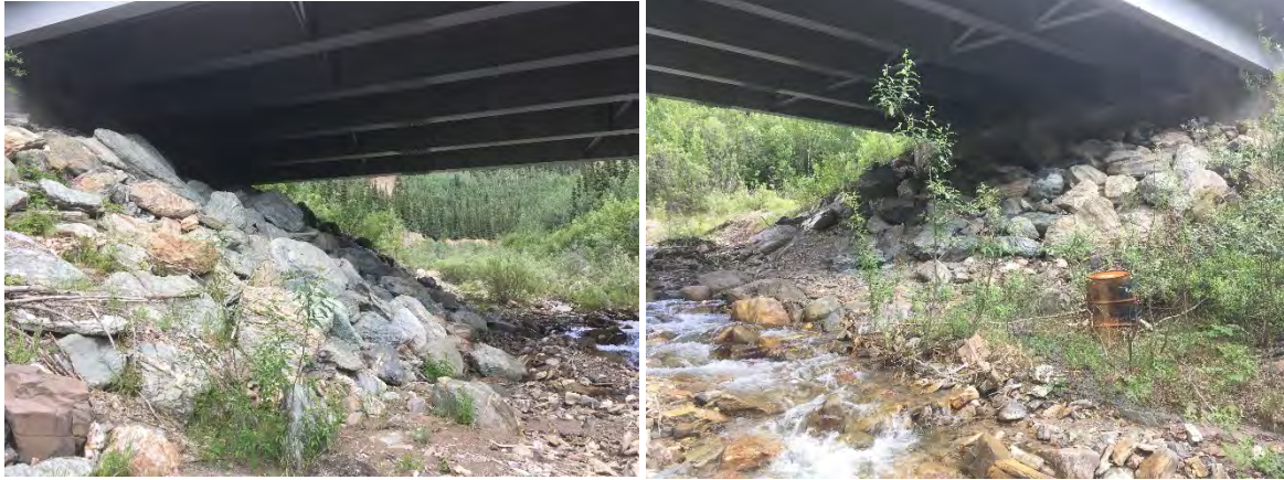
Figure 24. Looking Upstream, Left Abutment and Right Abutment
