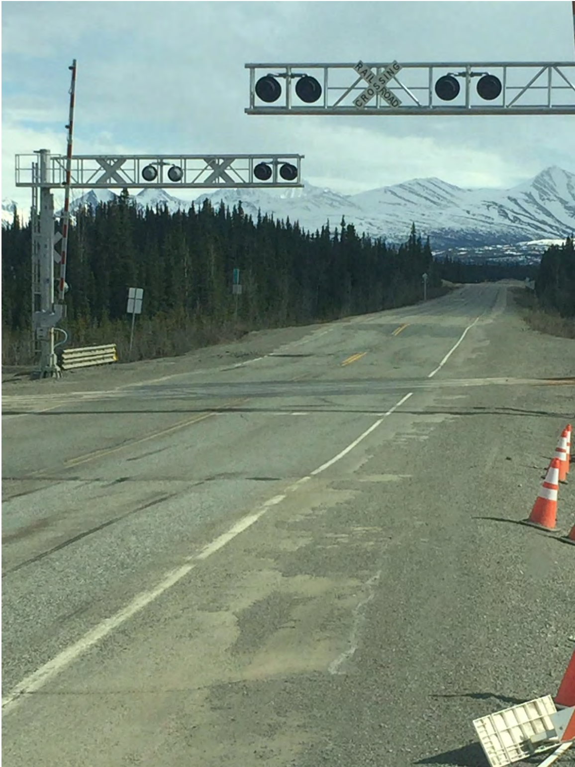
Figure 9 – Problematic Railroad Crossing at MP 235 of the Parks Highway
