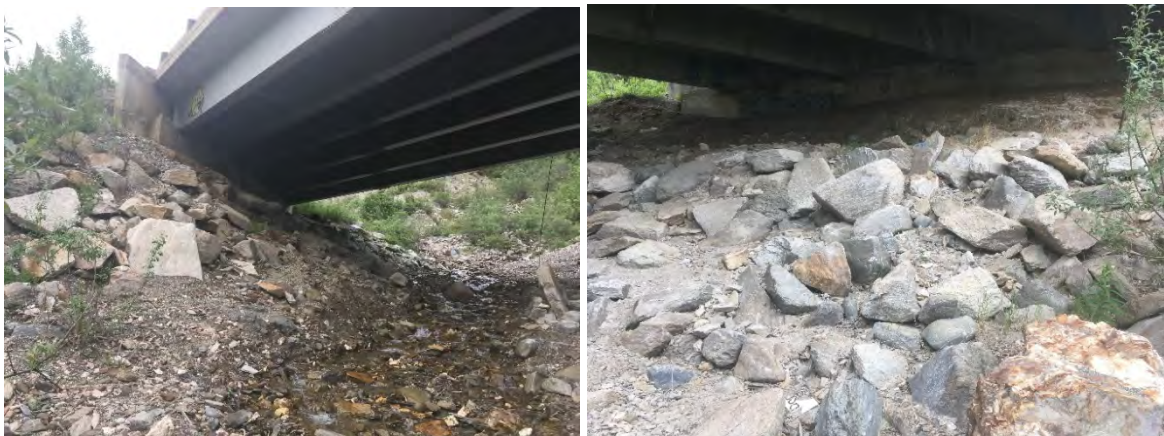
Figure 19. Looking Upstream, At Left Abutment and Right Abutment
