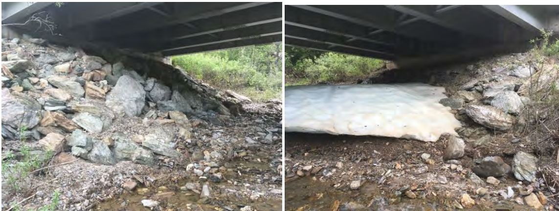
Figure 27. Looking Upstream, Left and Right Abutment
