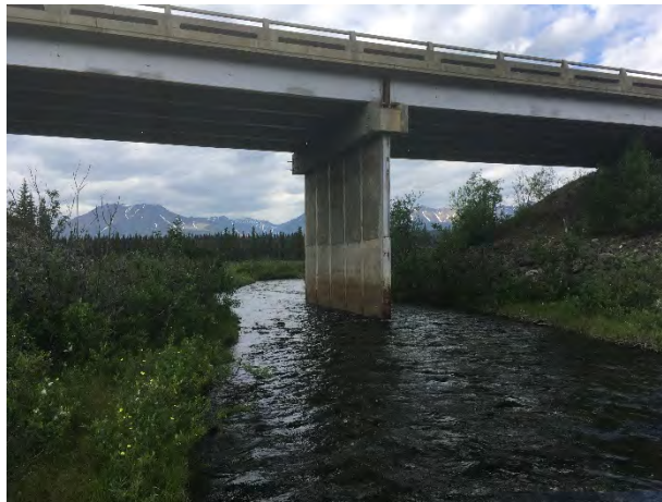
Figure 2. Pass Creek Bridge (BR 0293) Upstream Looking Downstream
