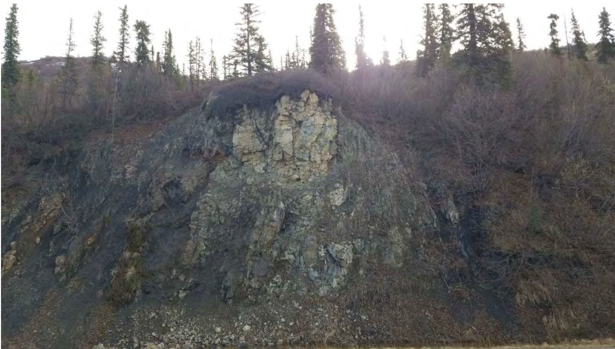
Rockfall near MP 212
