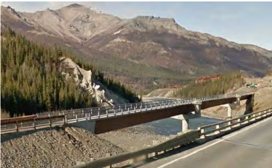
Non-motorized facility solution #3: pedestrian bridge
