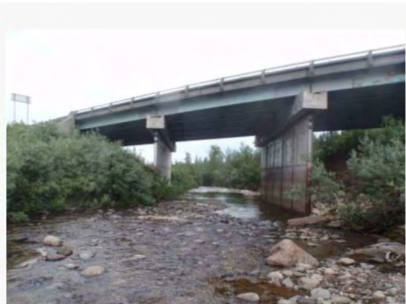
Panguingue Creek Bridge
