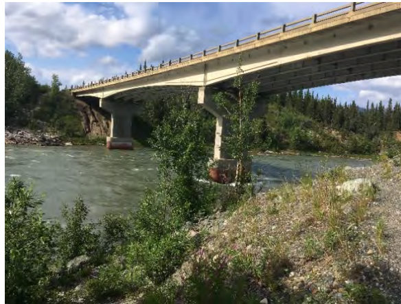
Figure 12. Nenana River Bridge (BR 0694), Downstream Looking Upstream
