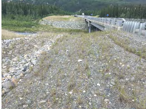
Figure 63. Typical Riprap Roadside Ditch Looking Toward Riley Creek
