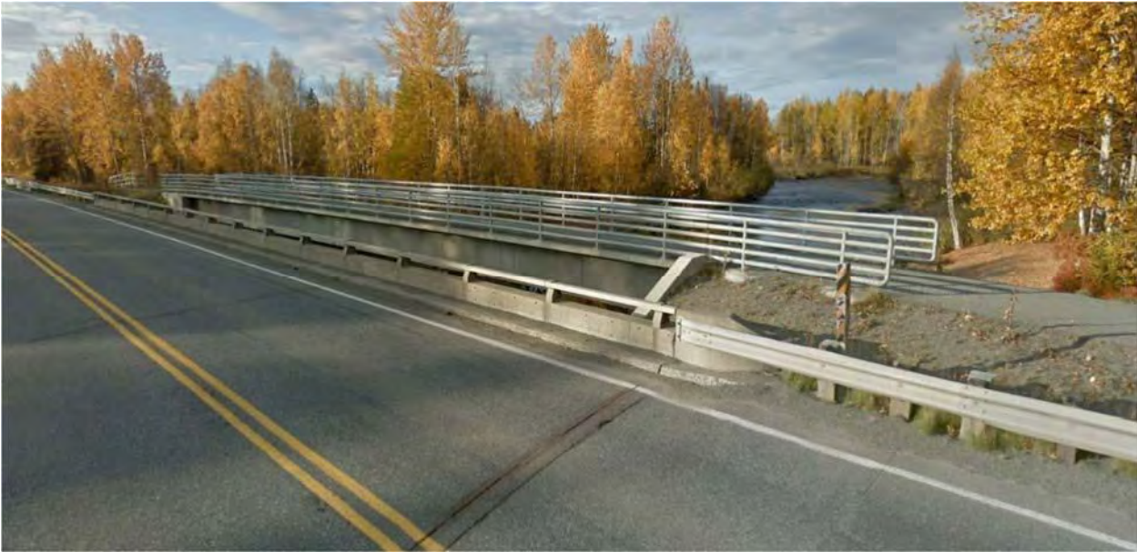
This is an example of a pedestrian bridge that could be built.
