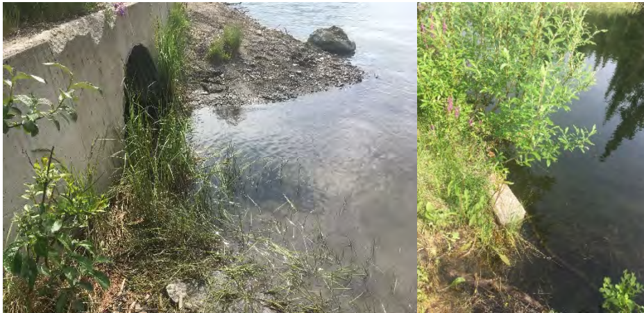
Figure 55. Culvert Just North of MP 222, Downstream Looking South, Upstream Looking North
