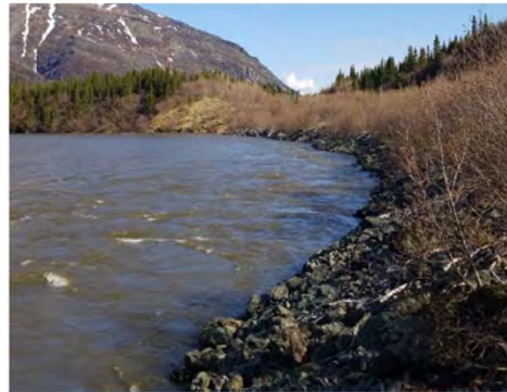
Existing erosion protection along Nenana River (~MP 219)
