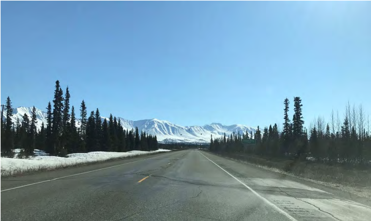
Roadway condition: pavement cracks (MP 211)
