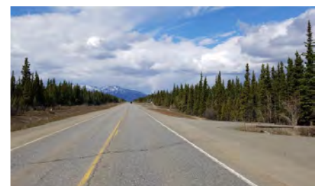
Several stretches along the corridor contain numerous driveways directly connecting to the highway, such as this photo depicting driveways near MP 229
