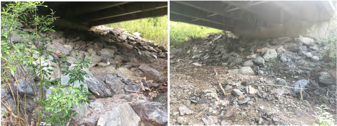
Figure 31. Looking Upstream, Left and Right Abutment
