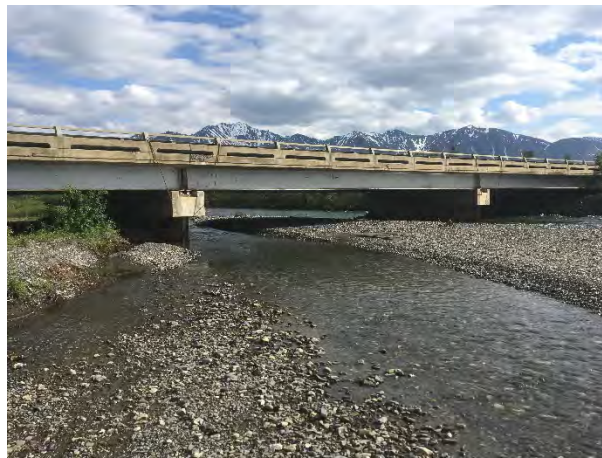
Figure 4. Jack River Bridge (BR 0293) Downstream Looking Upstream
