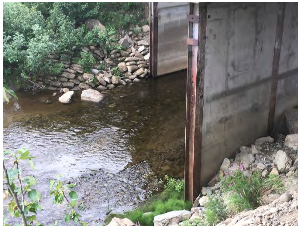
Figure 42. Panguingue Bridge (BR 0313), Downstream Looking Upstream and South
