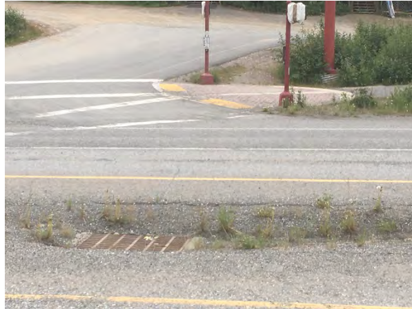
Figure 56. Storm Drain Median Inlet Near MP 238.6
