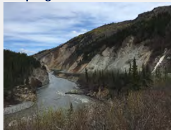
The highway is constrained by areas of slope instability and erosion by the river in the Nenana Canyon (MP 239-241)
