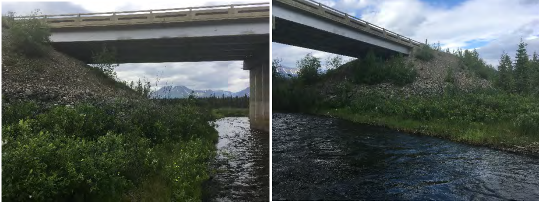
Figure 3. Looking Upstream, Left and Right Abutments
