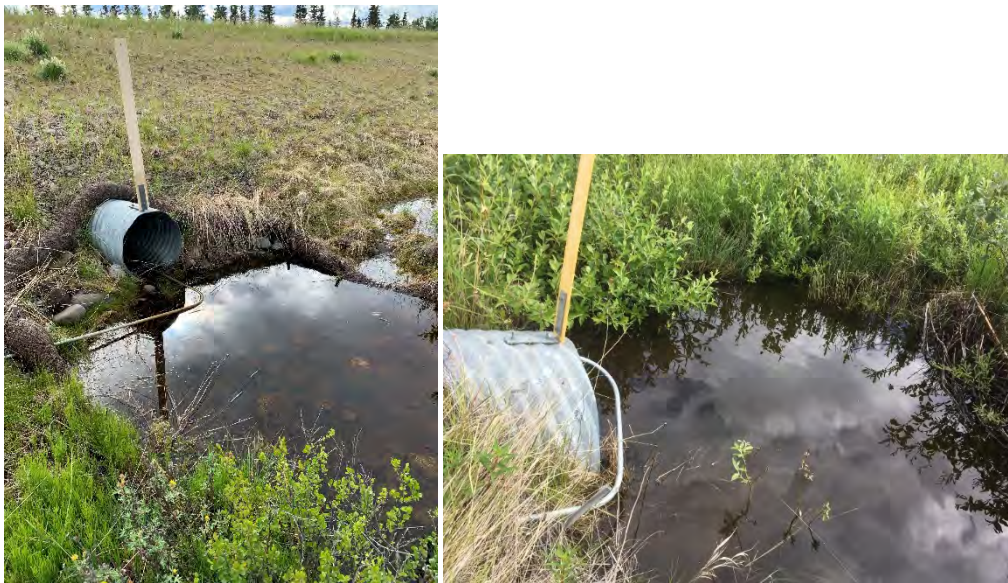
Figure 50. Upstream End of Culvert (West Looking East): Downstream End of Culvert
