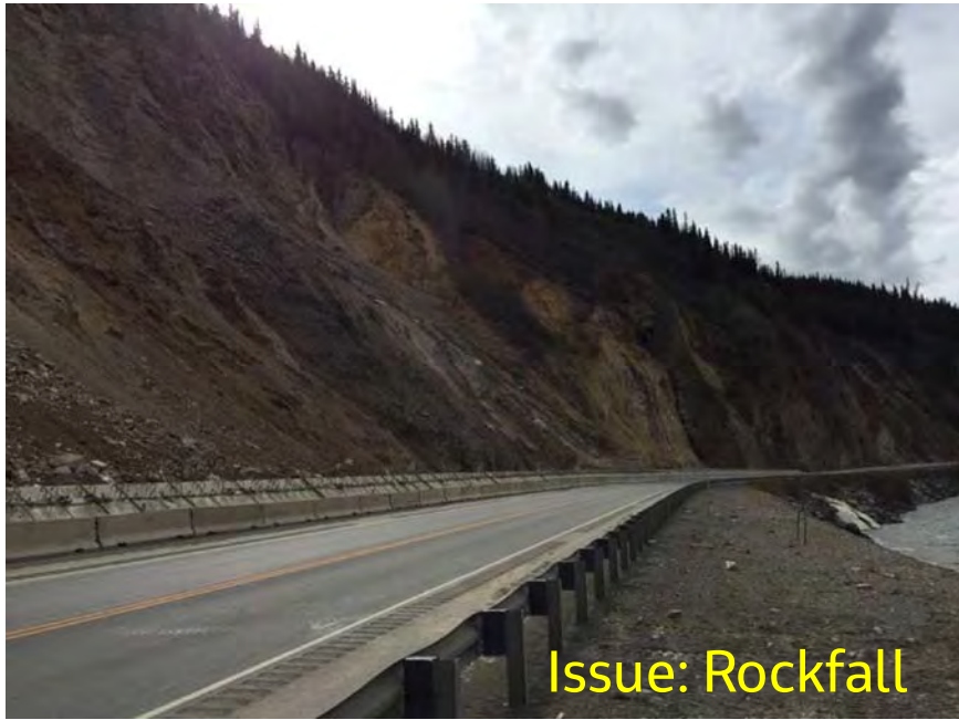
MP 239.6 Nenana Canyon rockslide area with robust concrete barrier
