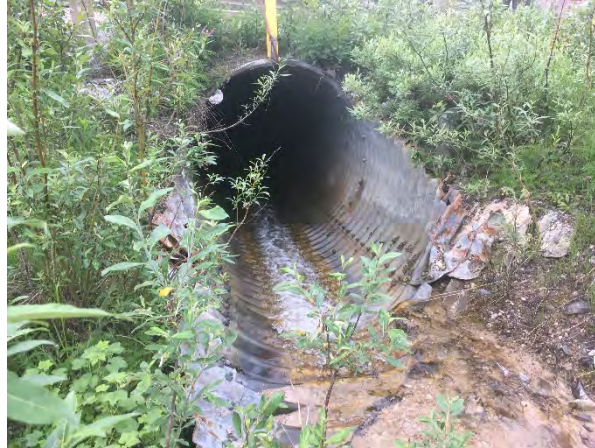
Figure 20. Junco Creek Cross Culvert, Upstream Looking Downstream
