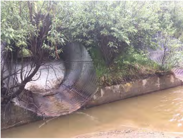
Slate Creek cross culverts (near MP 257.8)
