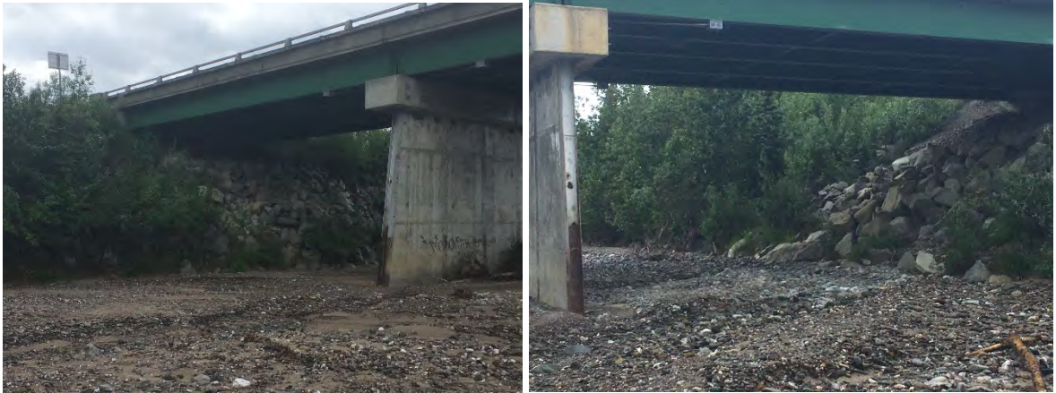
Figure 41. Looking Upstream, Left and Right Abutment
