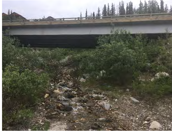
Figure 18. Kingfisher Creek Bridge (BR 0697), Downstream Looking Upstream
