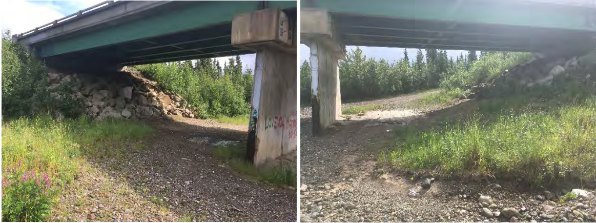
Figure 39. Looking Downstream, Left and Right Abutment
