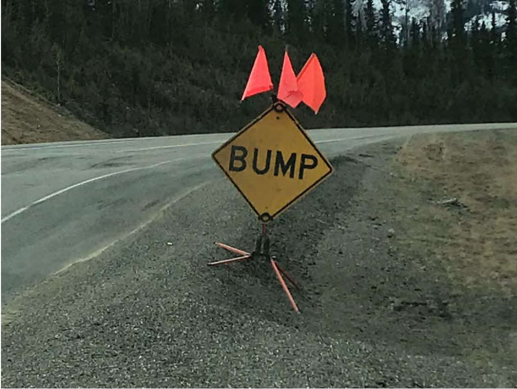
Figure 7 - Additional photo of bumpy section near MP 232.5
