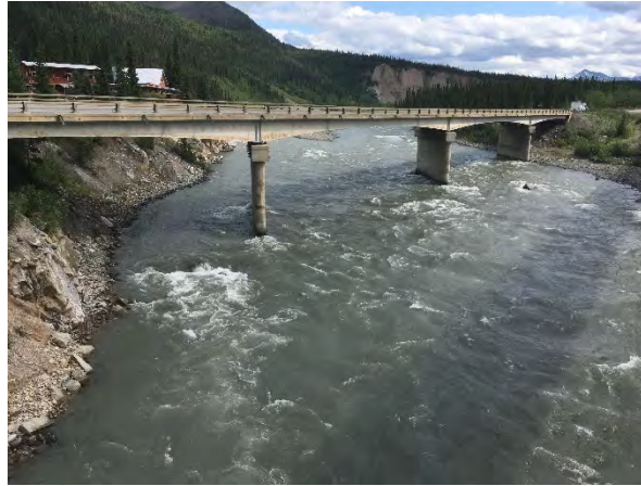
Figure 16. Nenana River Bridge (BR 1147), Downstream Looking Upstream
