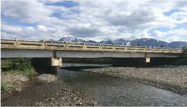
Jack River Bridge, downstream looking upstream
