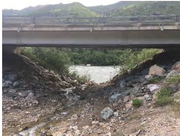
Figure 21. Iceworm Gulch Bridge (BR 1146), Upstream Looking Downstream
