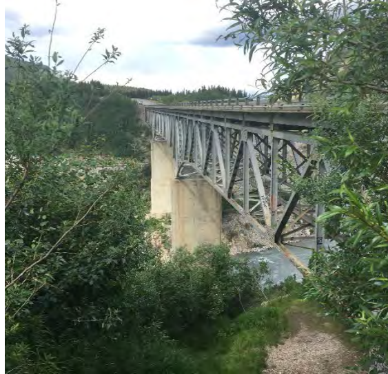
Figure 33. Nenana River Bridge (BR 1143), Downstream Looking Upstream and North
