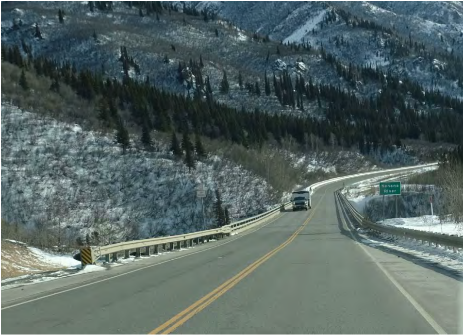
Nenana River bridge, located north of Nenana Canyon near MP 243, is one of several “pinch points” in the corridor for pedestrians: the highway shoulders are narrow.
