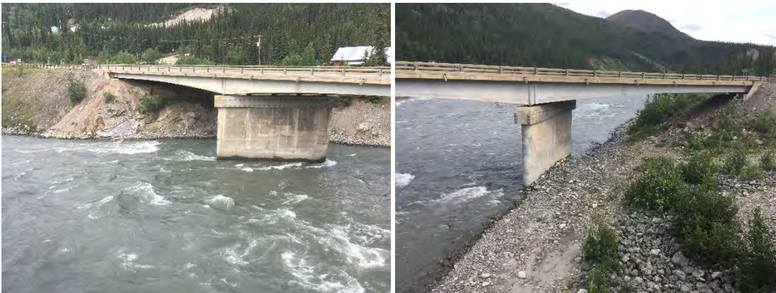
Figure 17. Looking Upstream, At Left Abutment and Right Abutment
