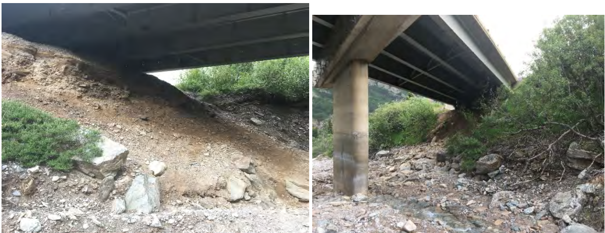
Figure 36. Looking Downstream, Left and Right Abutment
