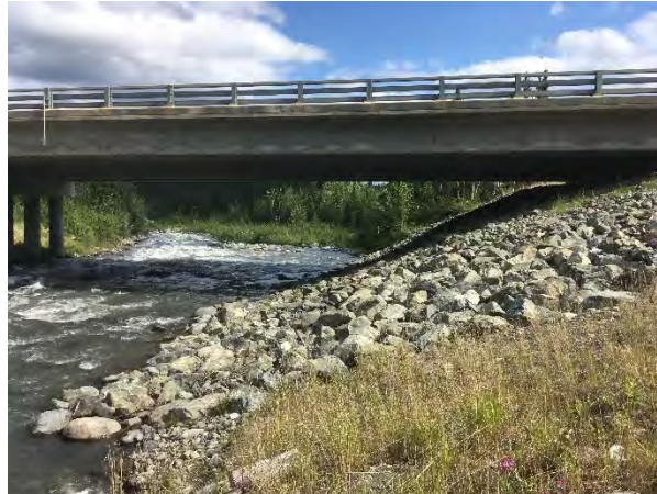
Figure 14. Riley Creek Bridge (BR 0695), Upstream Looking Downstream at Right Abutment
