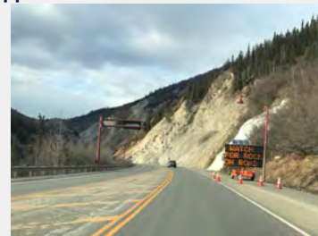
Rockfall hazards (MP 239-241)
