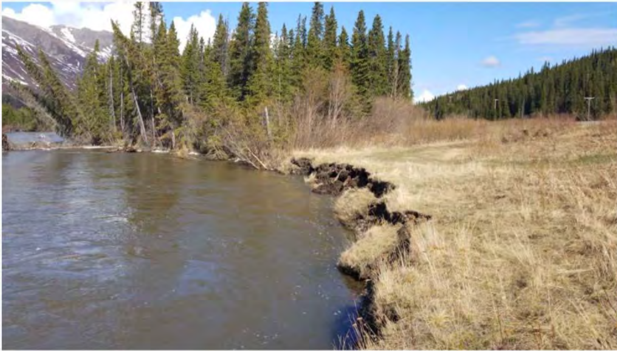
Embankment concerns near MP 222
