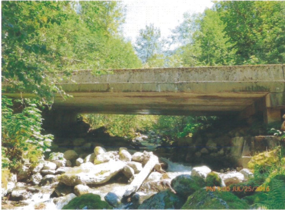
BEDAL CREEK BRIDGE-FLTPS1 OVER BEDAL CREEK Snohomish County, Washington
