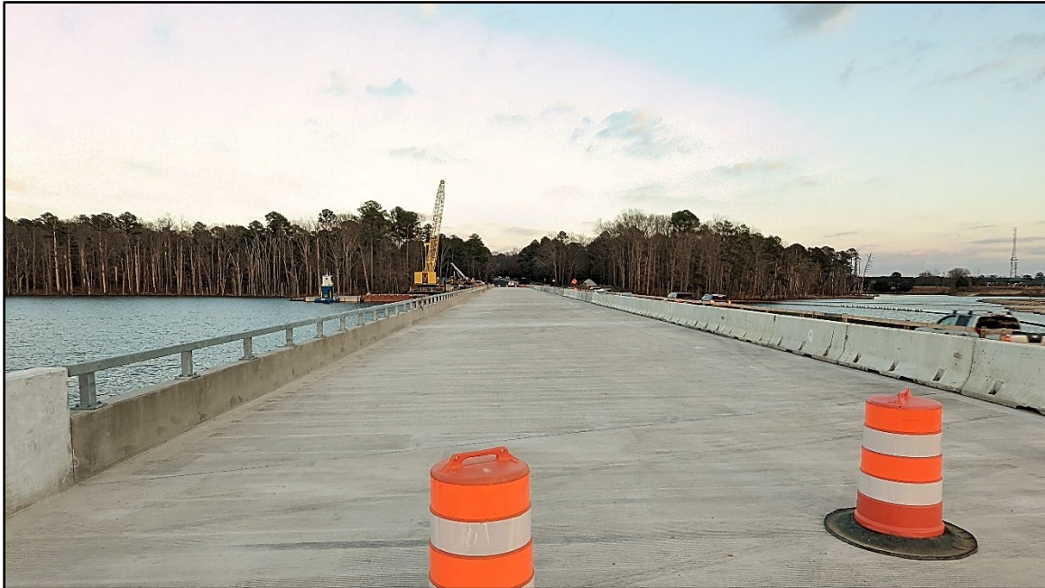
Westbound Span of New Bridge (Looking East)
