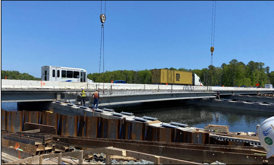
Girder Delivery and Placement on Eastbound Span #2 (Looking Northeast)
