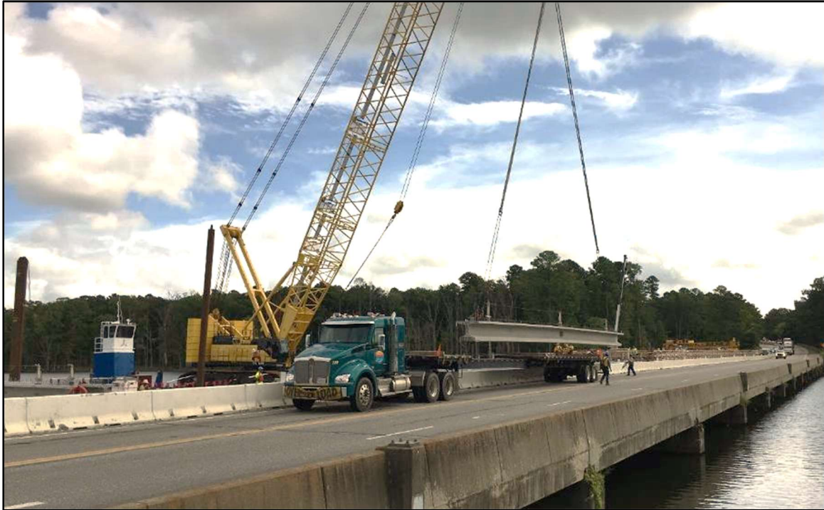
Girder Delivery and Placement on Westbound Span (Looking Northeast)
