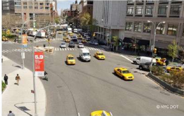
Figure 11. Lincoln Center Bowtie Street improvements included reduced lane width and turn calming.
