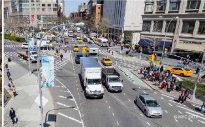
Figure 11. Lincoln Center Bowtie Street improvements included reduced lane width and turn calming.
