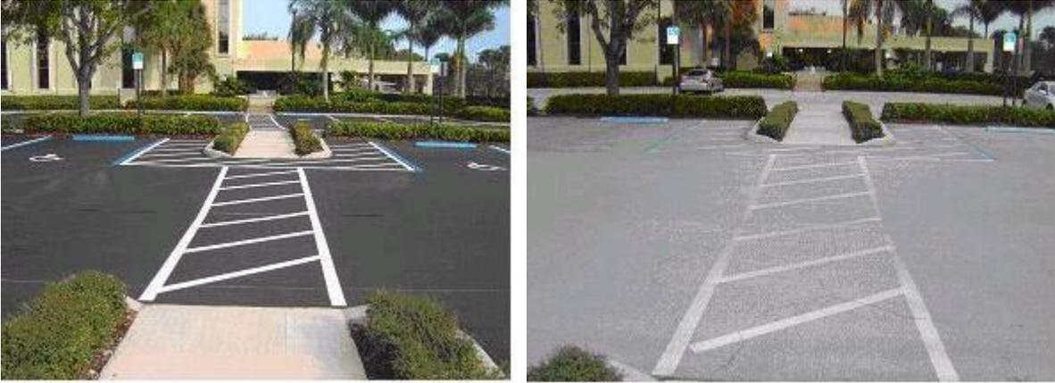
*The panel to the left shows newly painted crosswalk pavement markings. Notice the difference in contrast between the markings and the new, dark pavement surface. The panel to the right shows aged crosswalk markings. Notice the reduction in contrast between the markings and the lighter pavement surface.*
