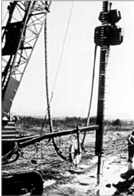
Figure 36. Wick drains being installed at an embankment on soft clay site.
