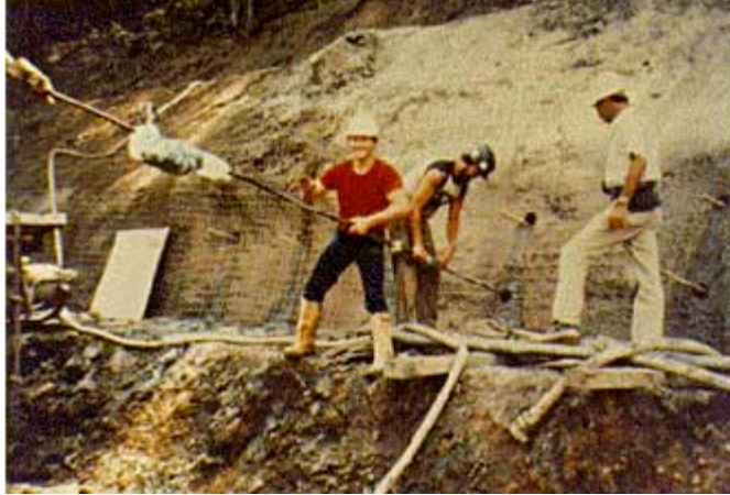
FIGURE 33. Installation of instrumented soil nail at Cumberland Gap site.
