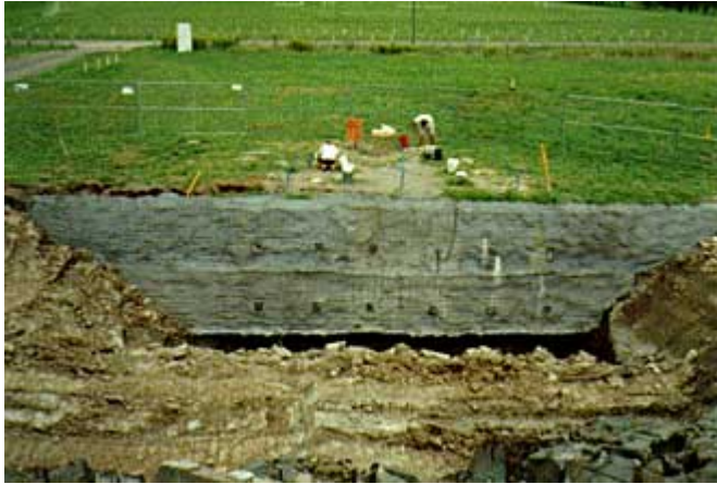
FIGURE 34. Failed soil nail wall due to undercutting.
