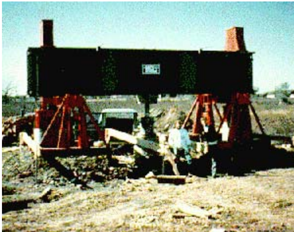
FIGURE 18. Vertical load test of defective drilled shaft.
