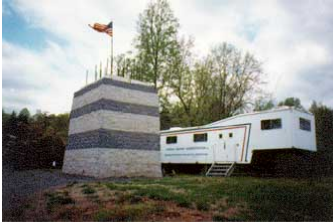
FIGURE 29. Geosynthetic reinforced soil support pier.
