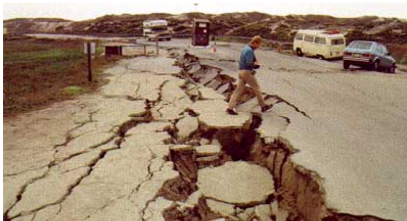
FIGURE 47. Liquefaction damage due to Loma Prieta earthquake.
