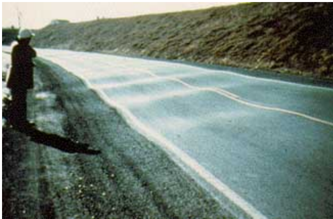
FIGURE 40. Pavement damage due to frost heave.
