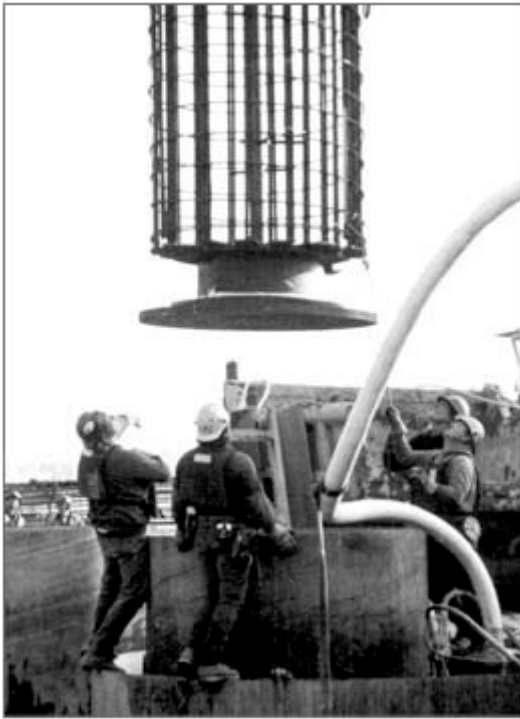
Figure 25. Osterberg load cell ready for placement in drilled shaft.
