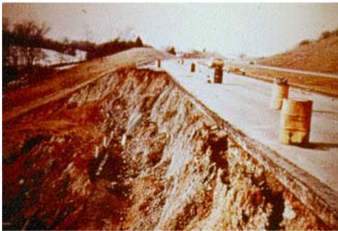
FIGURE 41. Shale embankment failure on I-64 in Indiana.
