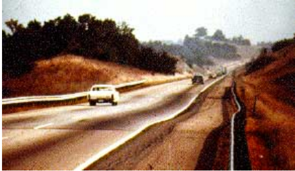
FIGURE 37. Pavement damage due to expansive subgrade soils.
