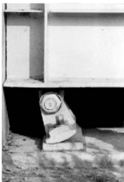
FIGURE 2. Bridge girder jammed against abutment and excessive rocker tilt.
