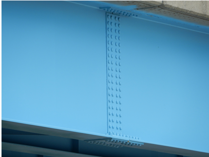
Figure 44. Photo. Example of view of girder splice plate.
