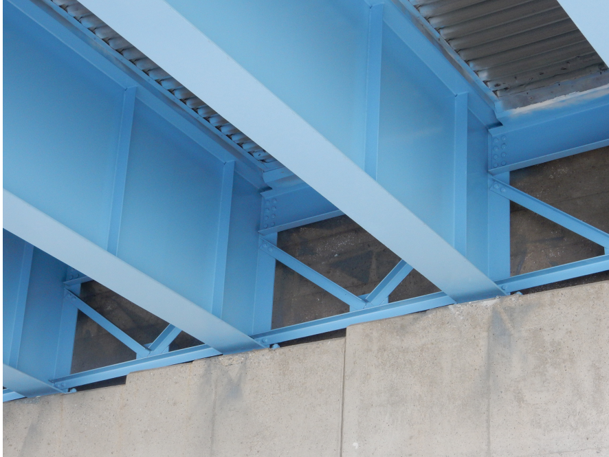
Figure 42. Photo. Example of view of bearing location.
