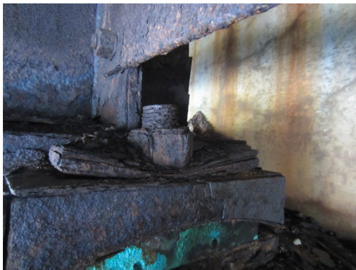
Figure 45. Photo. Example of closeup view of lateral bracing to girder connection.
