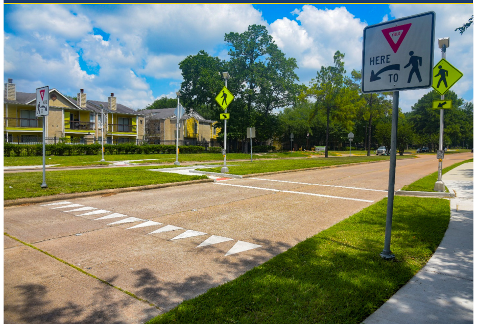
Figure 1. Photo. Example of LED-Em treatment on a four-lane divided street.
