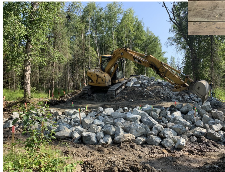
Left: Placement of Riprap around the South Fork Main Bridge abutment.
