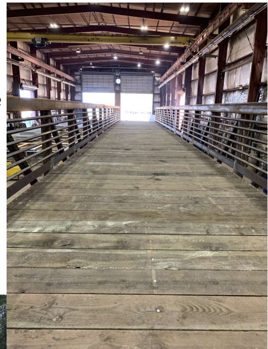
Right: South Fork Main Bridge Inspection
