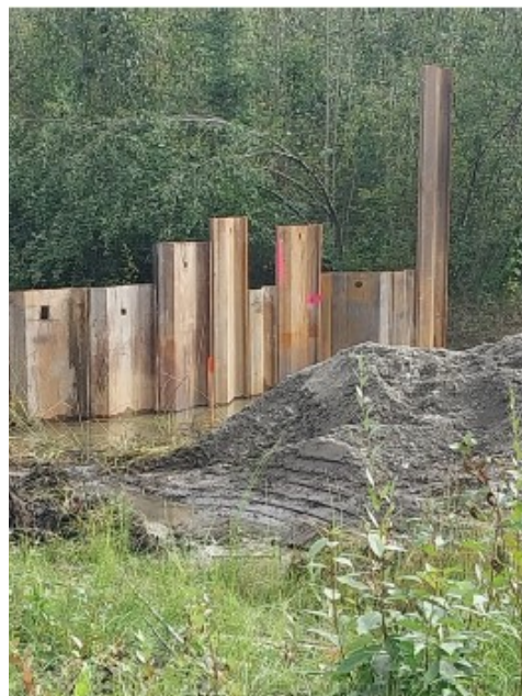
Left: Sheet pile dam.
