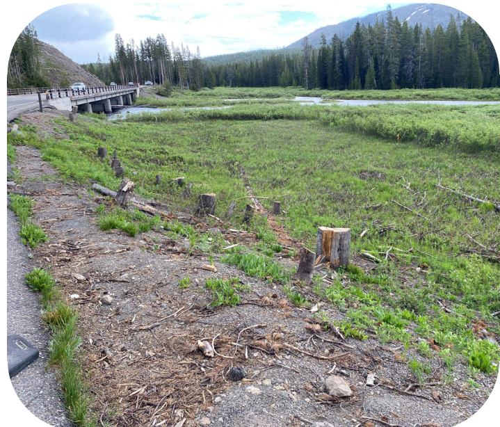
Project right after clearing and before wetland topsoil was stripped and conserved along disturbance.
