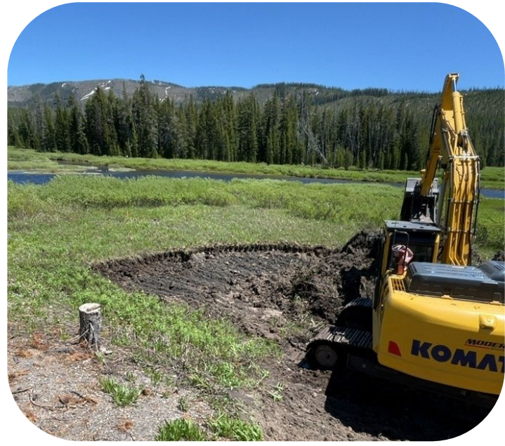
Project right during the strip and conserving of wetland topsoil
