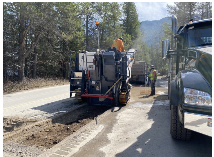
Milling existing trenches to prep for paving on Apgar Loop Road.
