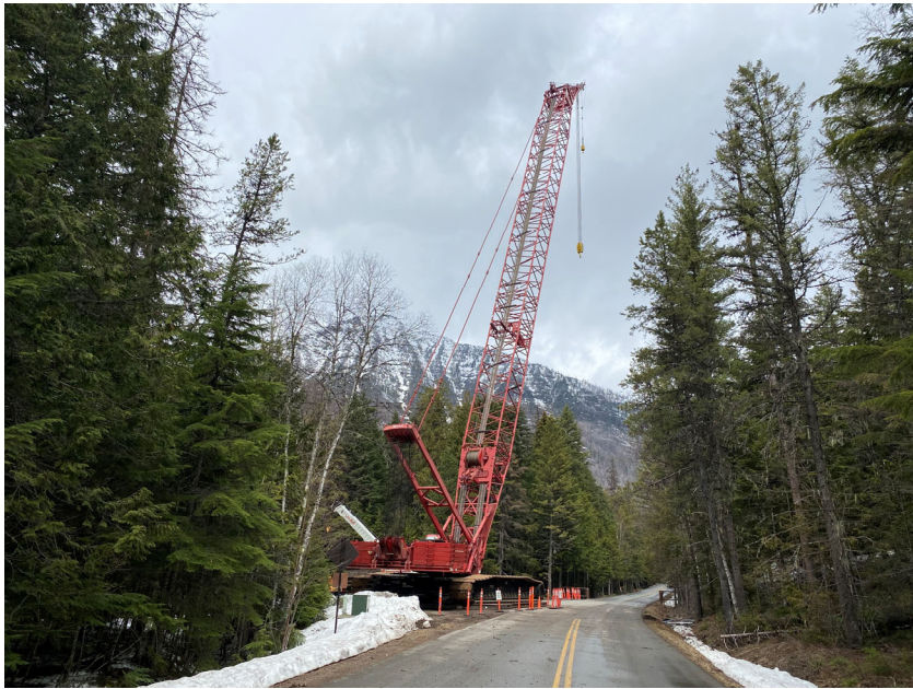
440 Ton Manitowoc crane 30' wide from track to track 175' boom length
