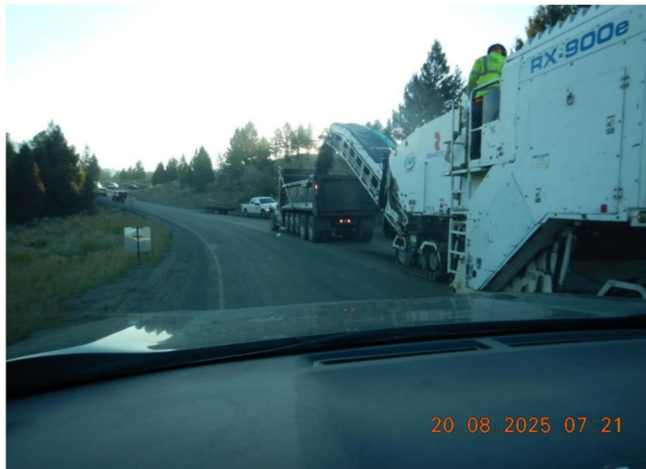
Milling at East Bridge end
