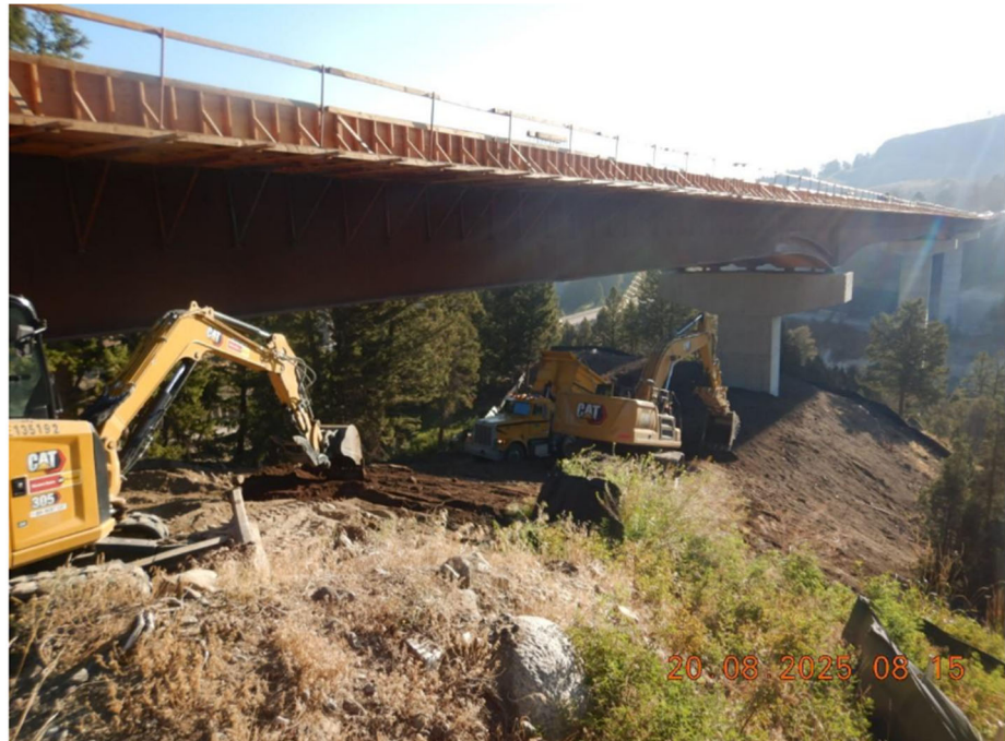
Embankment and Topsoil Abut 1 to Pier 1
