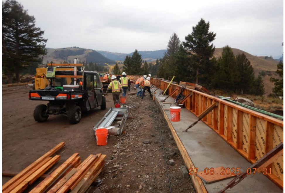
Guardwall forms for corewall Station 144+50-146+50LT
