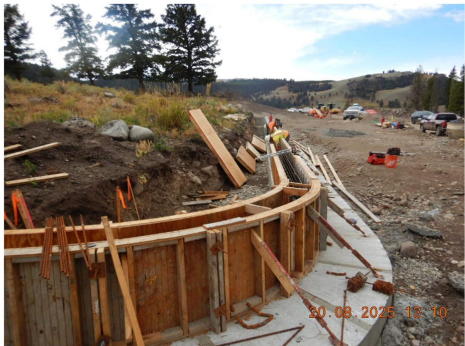
Bridge and Canyon Overlook guardwall
