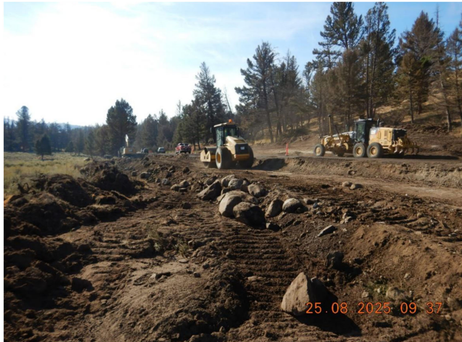
Earthwork near station 161
