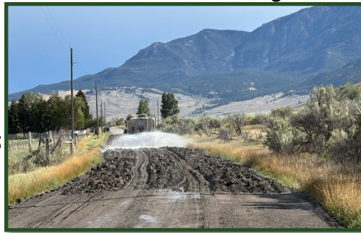
Processing Roadbed Material
