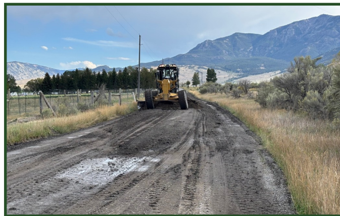
Processing Roadbed Material
