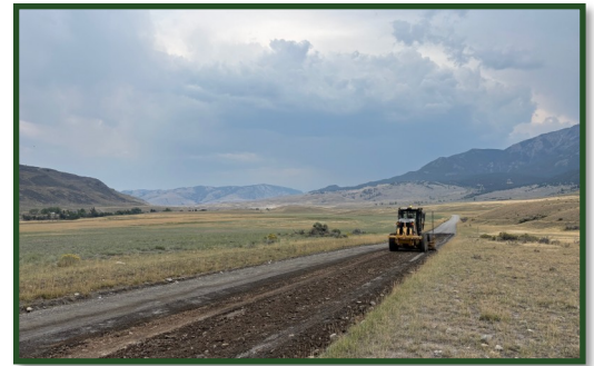
Processing Roadbed Material
