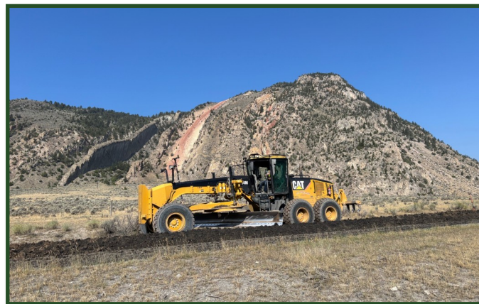
Processing Roadbed Material
