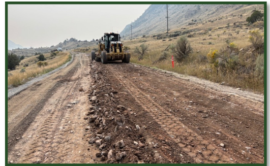
Processing Roadbed Material
