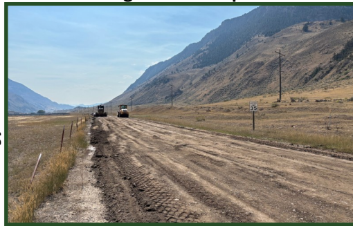
Processing Roadbed Material
