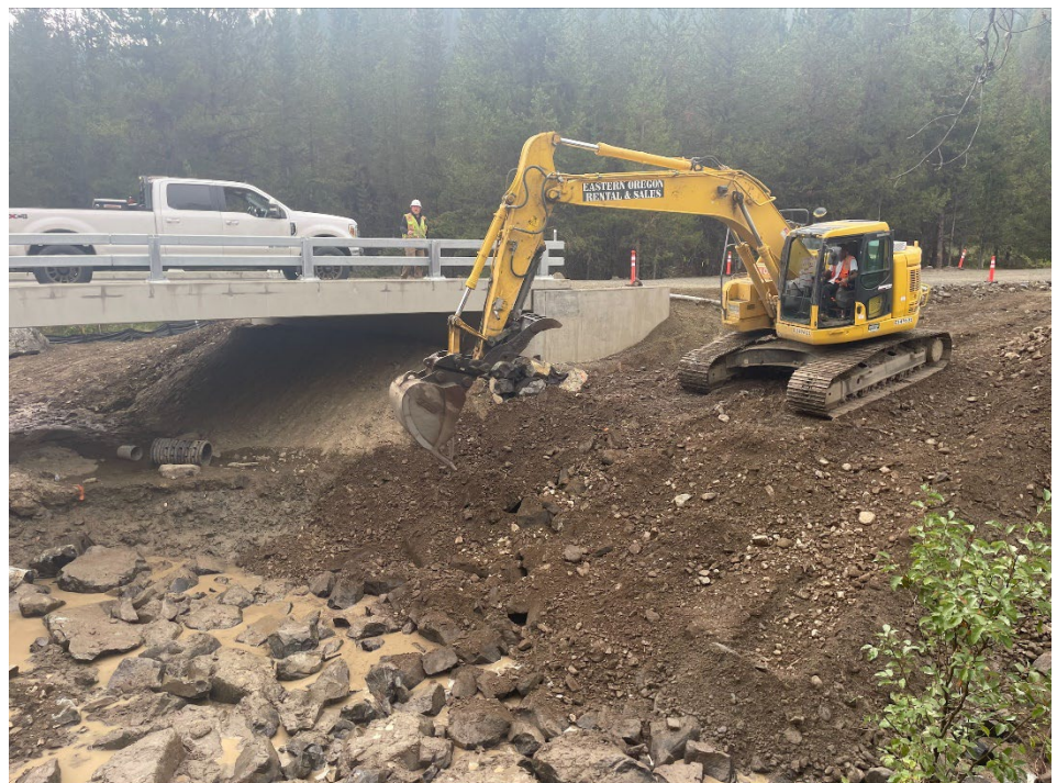
Bull Run #3, Bridge and Stream Work
