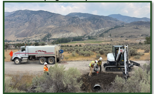
Culvert Installation
