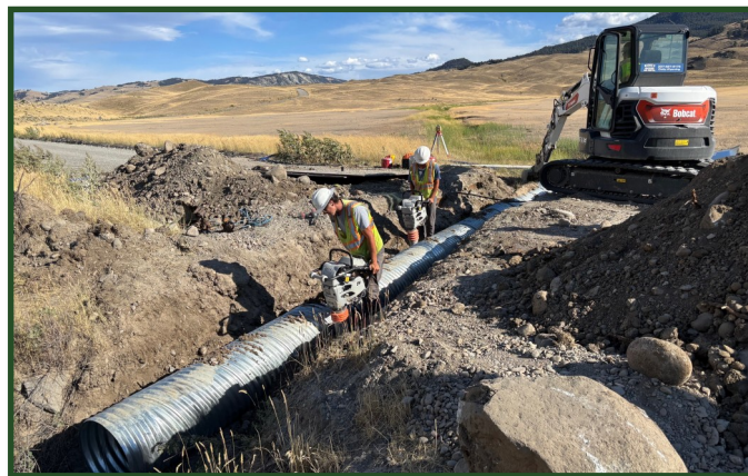
Culvert Installation
