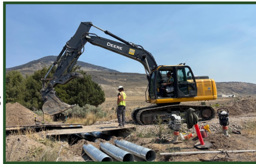
Culvert Installation
